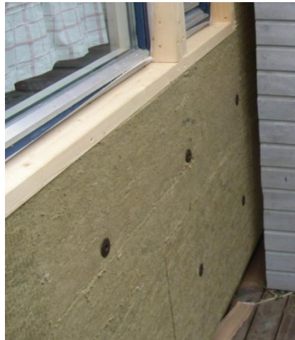
Figure 38. Refurbishment by TOBB in Trondheim 2010.
