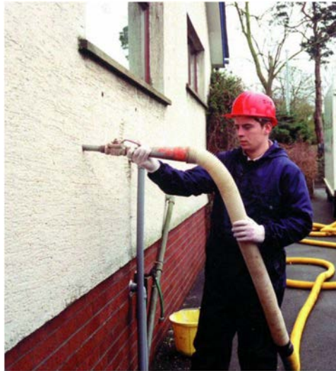
Figure 14. Installation of cavity insulation (EST 2007).
