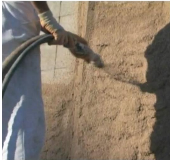
Figure 8. Applying insulating plaster (Protherm 2011).
