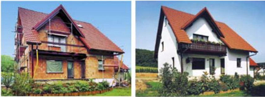
Figure 1. Façade before and after installing external thermal insulation (Rockwool).
