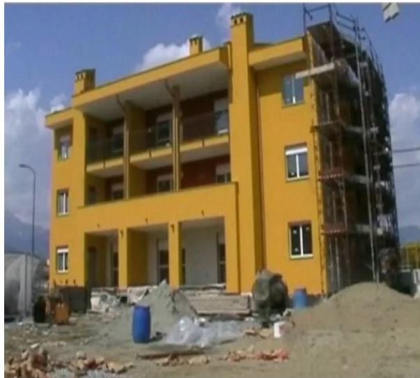
Figure 7. Insulating plaster finished with paint (Protherm 2011).
