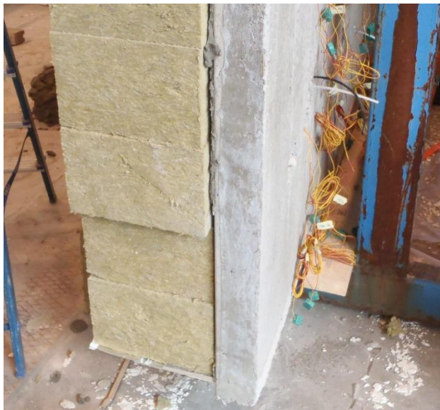
Figure 5. Concept T1b by VAHANEN, thermal plastered test wall at building phase.
