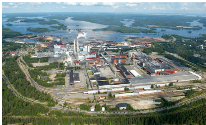
Figure 1. The facility of the UPM biorefinery is located in Lappeenranta, Finland, and will produce biodiesel from crude tall oil at UPM's Kaukas mill site.
