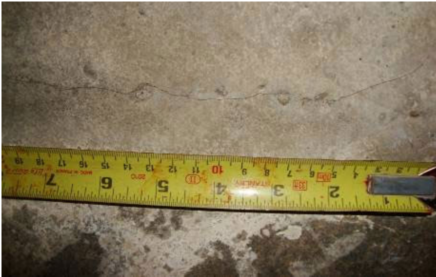
Figure 5. Observed micro-fracture at the repair interface.
