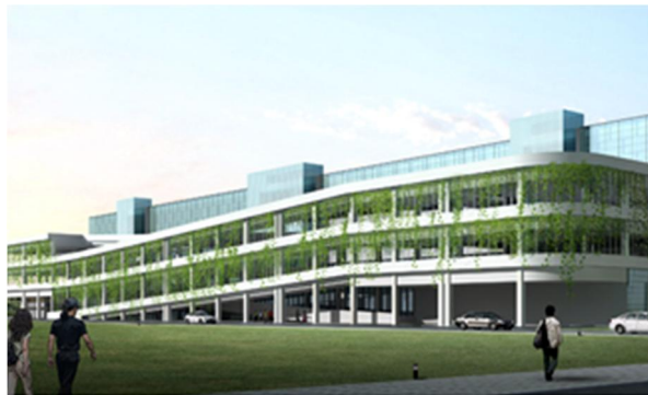
Figure 75. Vertical greening for the parking garage not only improves the building's appearance but also provides natural shading (Zhou 2012).
