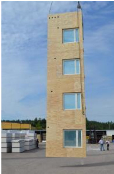
Figure 54. TES Energy Facade, Innova-project in Finland, Peltosaari (Lattke 2011).
