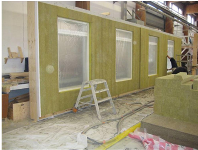
Figure 76. Prefabrication of the elements. (Picture: Ilpo Kouhia/VTT.)
