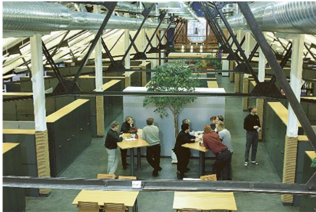
Figure 78. The only thing that was left of the old plywood factory was the original brick facade of the building with a special rose window and ten steel roof trusses. These were integrated into the new building as a reminder of the old architecture and construction tradition. (Photo: ARE Oy.)
