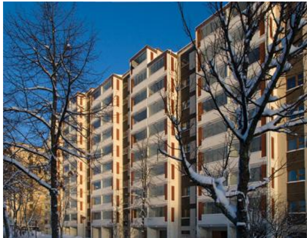
Figure 53. Glazed balconies in Finland (Lumon 2012).
