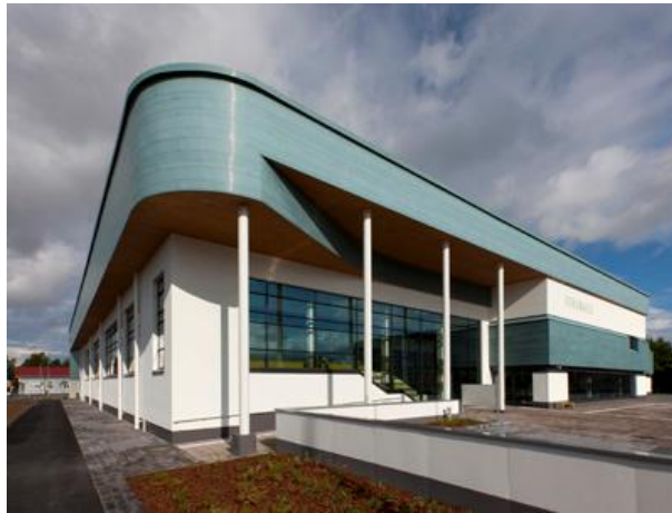
Figure 59. The water in the new swimming hall in Pori is heated with the façade-integrated Nordic Solar collectors. (Picture by Esa Kyyrö, source: Mörk 2011.)
