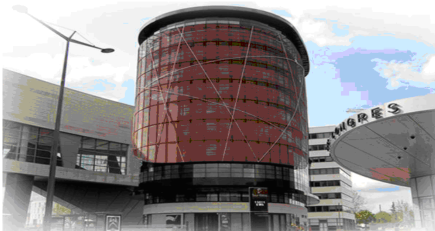
Figure 67. Elithis tower, France (Hernandez 2011).
