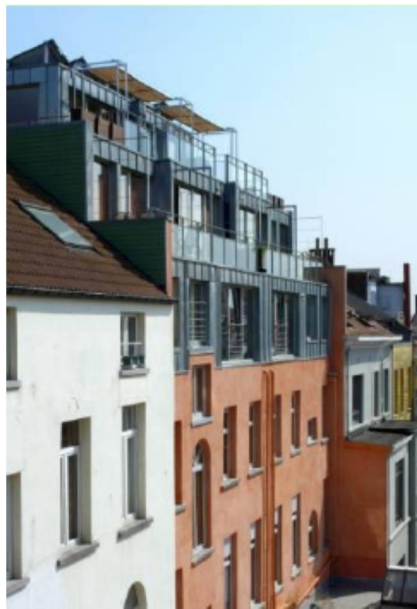
Figure 55. When the roof of this 19th century building in Brussels needed renovation, it was replaced with three additional wooden-structure floors (Desmedt et al. 2010).
