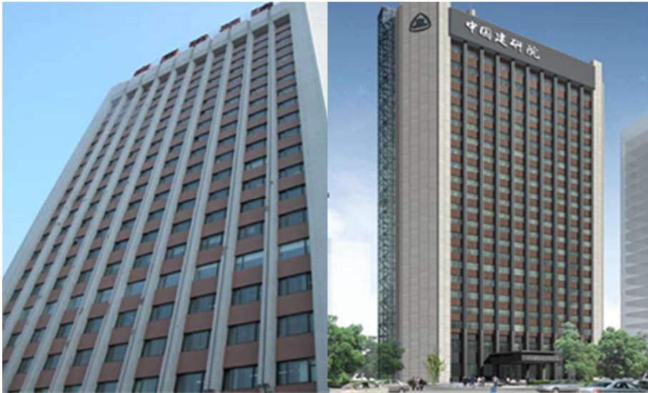
Figure 71. China Academy of Building Research before and after retrofit (Sjzu 2011).
