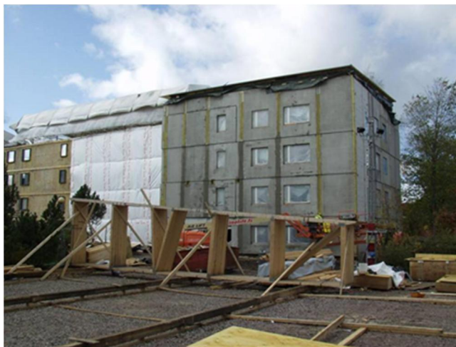
Figure 77. Installed TES elements. (Picture: Ilpo Kouhia/VTT.)
