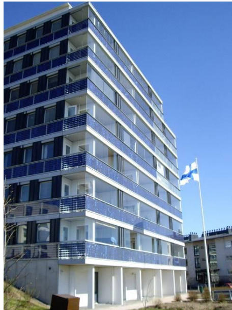
Figure 60. The façade of this residential building in the Viikki area in Helsinki is covered with PV-panels. (Photo: Christer Nyman.)
