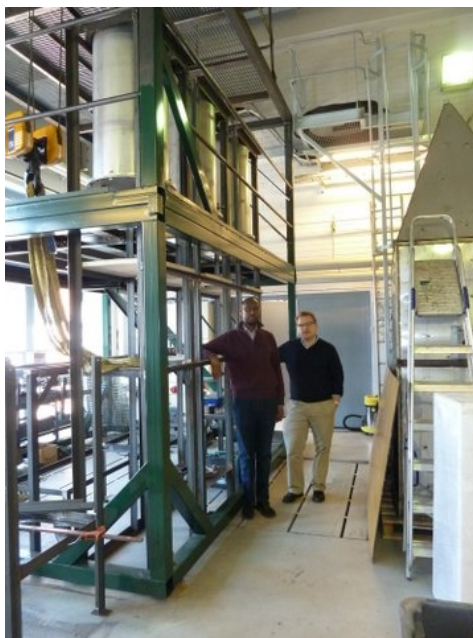
Figure 22. Pilot facility under construction at Aalto University.
