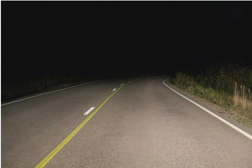
Figure C11. Site 4 with no delineator posts.
