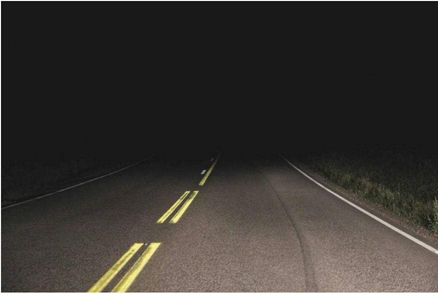
Figure C13. Site 5 with no delineator posts.
