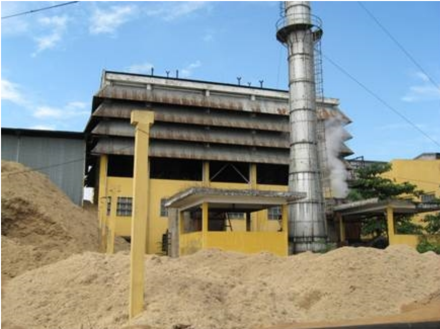
Figure 13. Power plant and bagasse storage at the backyard of the sugar mill in Ben Tre sugar mill (Photo by Arvo Leinonen).
