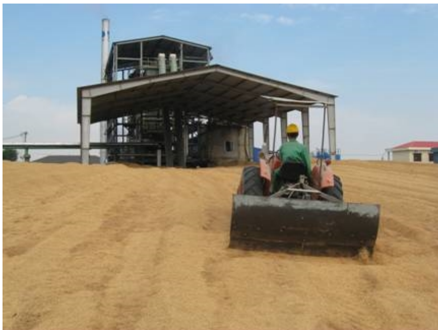
Figure 11. Rice husk storage at Dinh Hai power plant (Photo by Arvo Leinonen).
