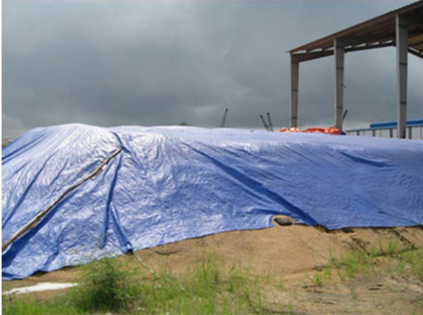
Figure 25. Buffer storage of rice husk at Dinh Hai steam power plant (Photo by Arvo Leinonen).
