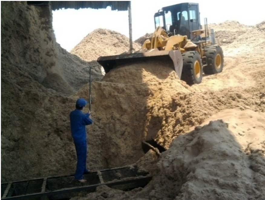
Figure 40. Feeding fuel to boilers (Photo by Duc Vu).
