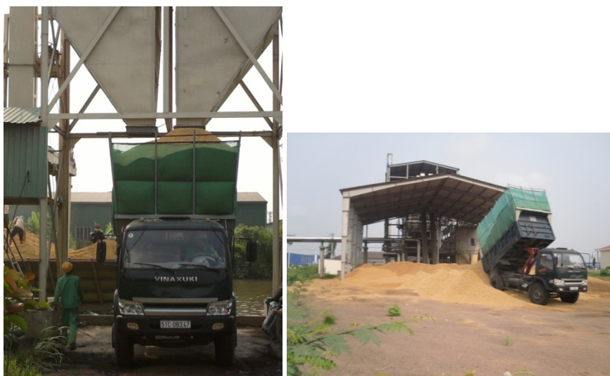
Figure 35. Transport of the rice husk from the river side into the covered storage at power plant (Photos by Duc Vu and Arvo Leinonen).
