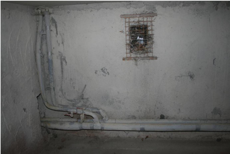
Figure 18. Standpipes rising from the cellar.
