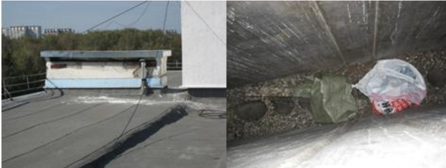
Figure 19. An exhaust unit in a roof.
