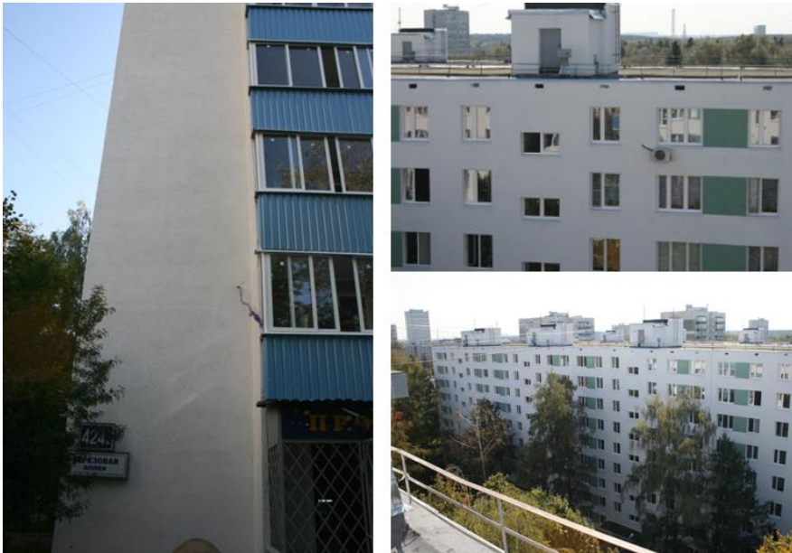
Figure 21. A renovated II-49 building.
