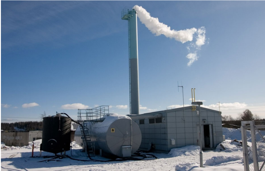
Figure 8.1. Fortum's district heating plant in Masala firing bio-oil in 2010.
