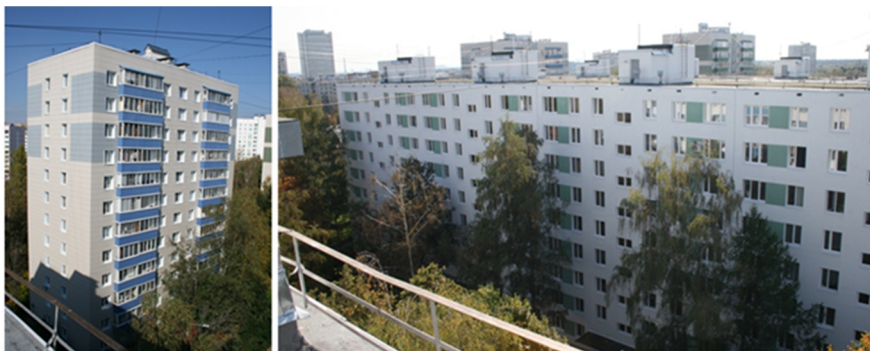
Figure 13. Apartment buildings in Zelenograd (Moscow) after capital repair in 2012 type II-18 (left) and II-49 (right).
