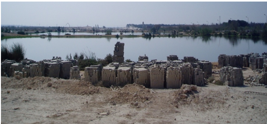
Figure 10. Picture of a waste stabilization pond (40,000 m 3 /d) for treatment of mixed industrial and domestic wastewater.
