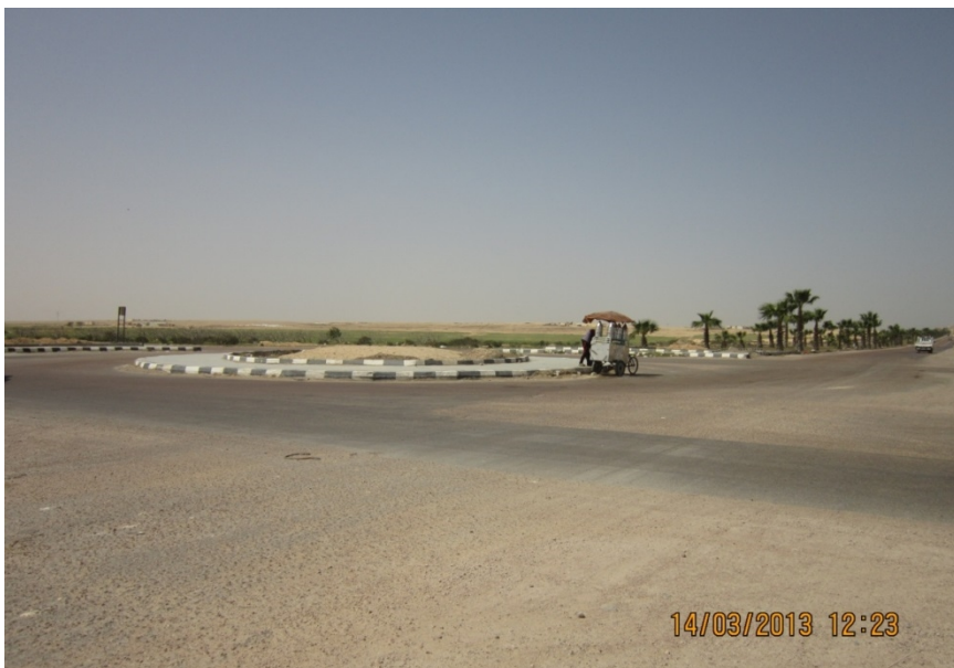
Figure 2/4. Ahmed Zewail Road and South Road Junction.
