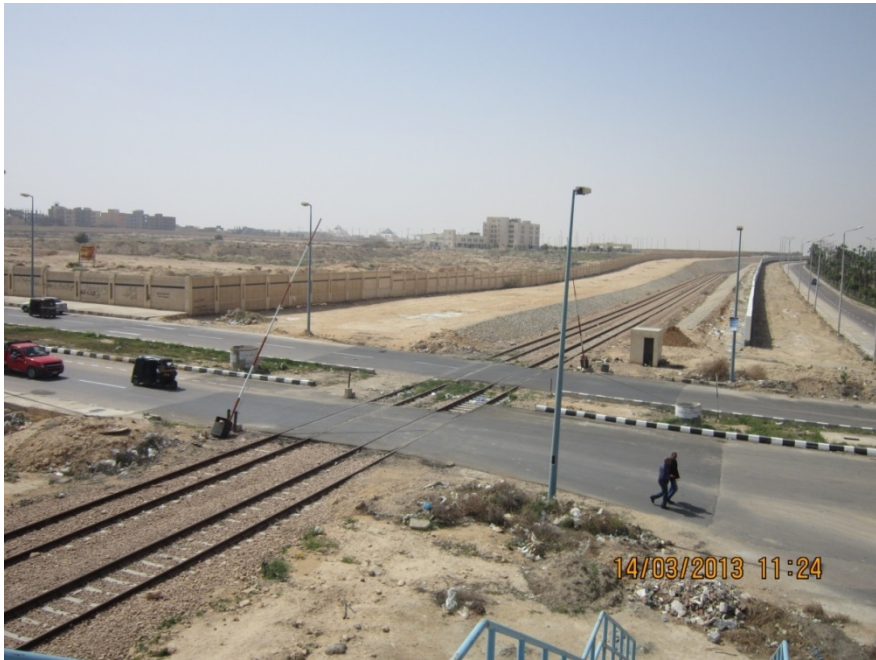
Figure 2/2. Court Street and Railway Line Junction.
