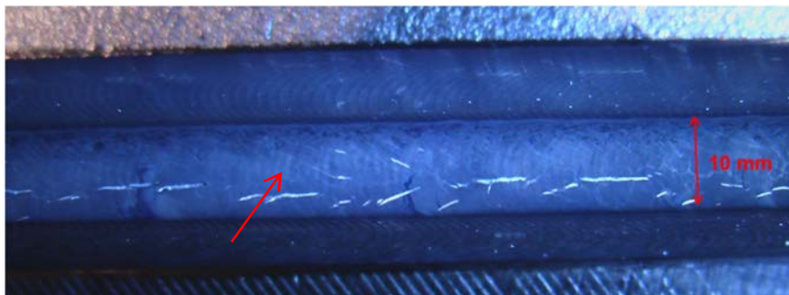
Figure 65. Hot cracking type weld defects in the surface of the first weld passes.
