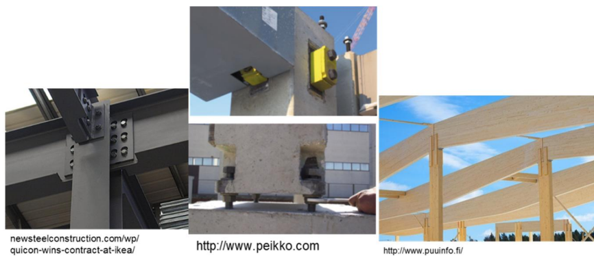
Figure 21. Design of demountable joints is important for re-use.
