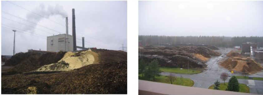
Figure 5. Storage sites of ready-made fuel and raw fuel material established in the close vicinity of usage sites secure the plant's fuel supply in all conditions.
