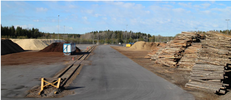
Figure 17. Söderenergi's feed-in terminal in Nykvarn, Sweden. Storage of ready-made fuel on the left, loading rail in the middle and buffer storage of stem wood on the right.
