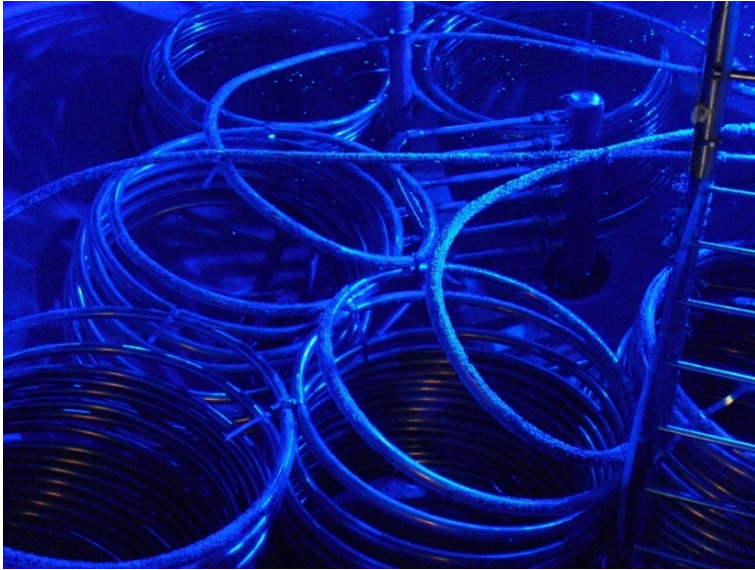
Figure 5. Condensation pipes used in the SBO experiments.
