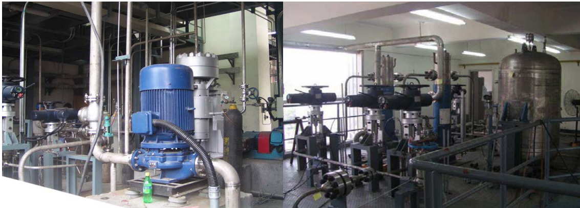
Figure 13. The SWAMUP thermal-hydraulic test facility at SJTU.
