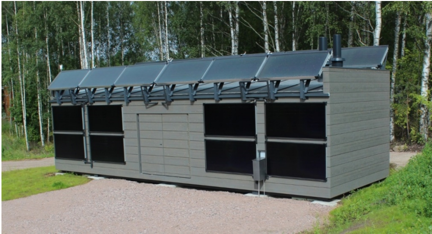
Figure 39. Savosolar collector installation (40 m 2 ) in Lappeenranta summer house fair (Savosolar, 2013).
