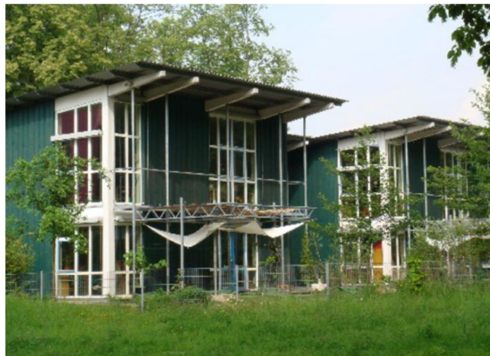
Figure 39. Residential houses in Vauban with solar shading solution integrated in the architectonics of the houses. (Åsa Hedman, VTT)
