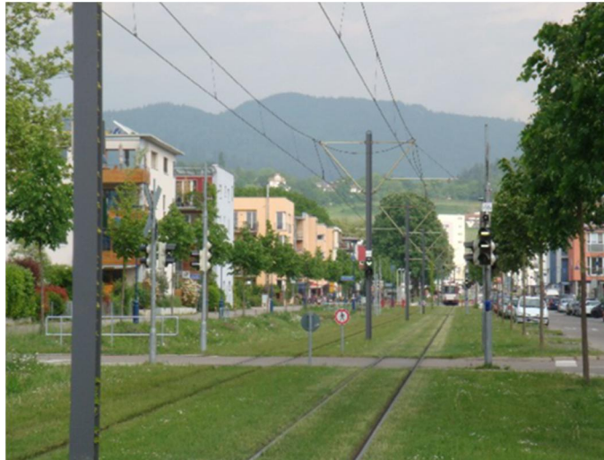
Figure 38. Tramline with grass lowering the noise level. (Åsa Hedman, VTT)
