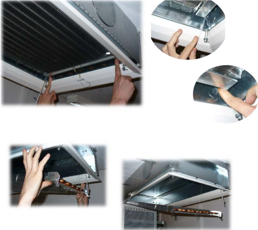
Figure 56. Active chilled beams to be installed in the ICU rooms.
