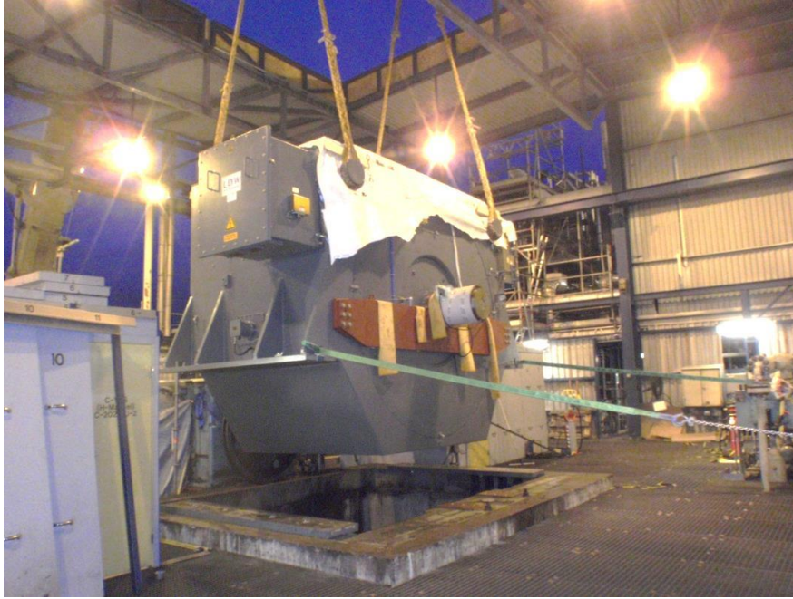
Photograph 2. Installation of new Hyper compressor E-motor [6].
