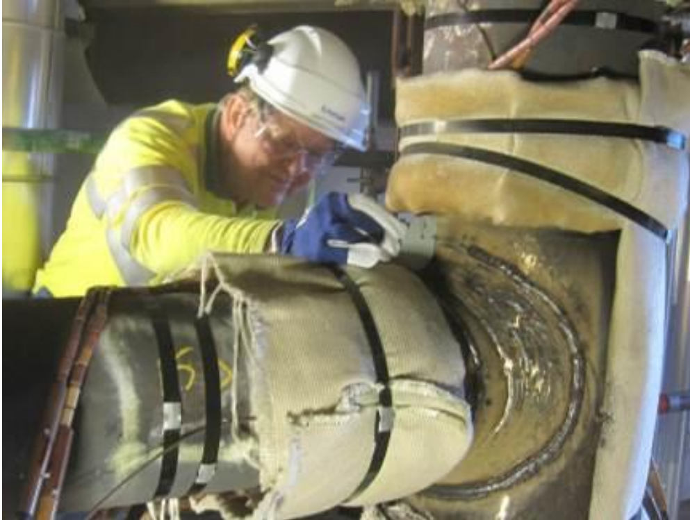
Figure 9. Repair welded branch to reduction valve (photo: Ville-Veikko Kylliäinen, Fortum).
