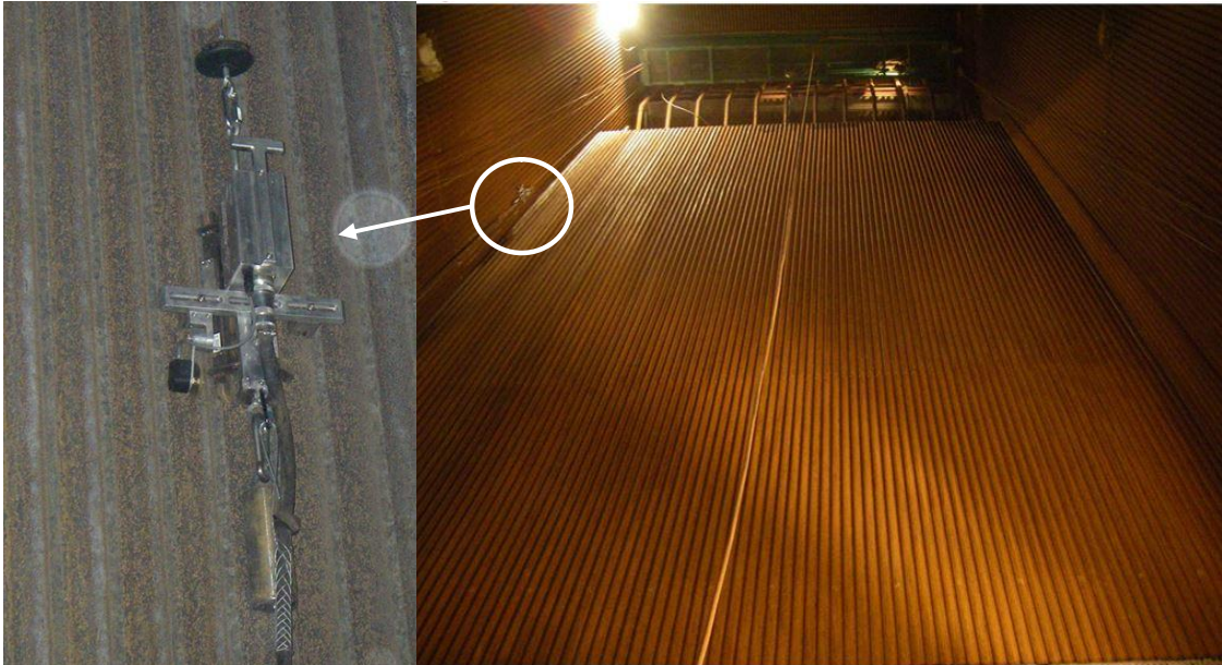
Figure 3. T-Scan crawler scanning the boiler membrane wall.
