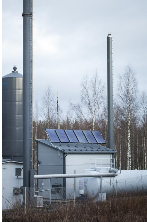
Figure 29. Savon Voima's pilot DH plant combining wood pellets, solar thermal and electric heater [94].
