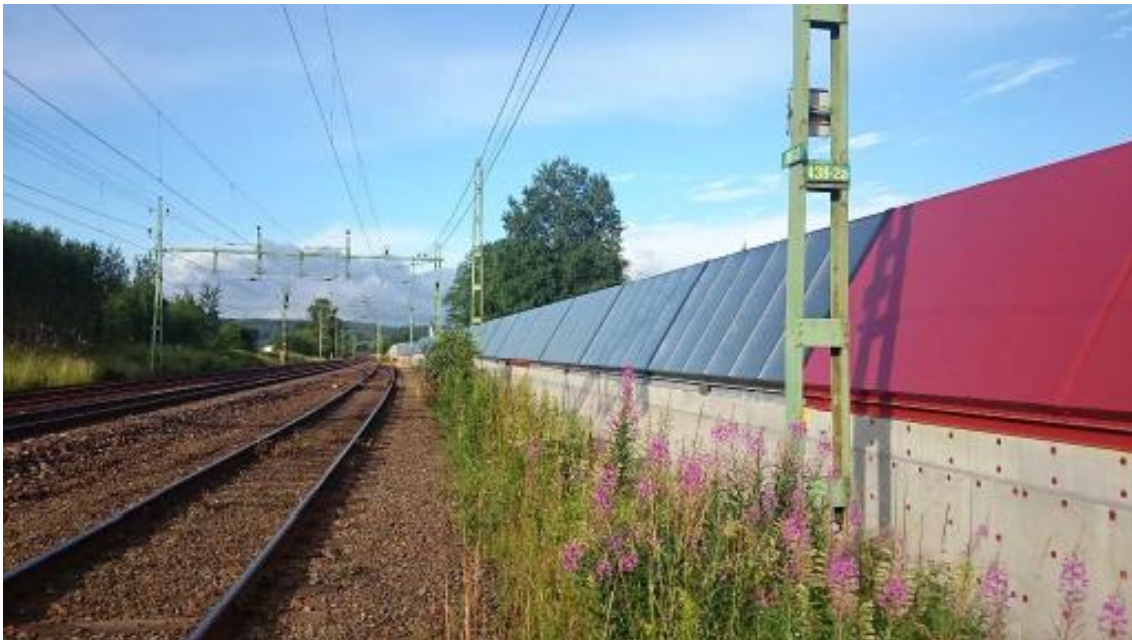
Figure 31. Solar heat collectors acting as a noise barrier in Lerum in Sweden [101].
