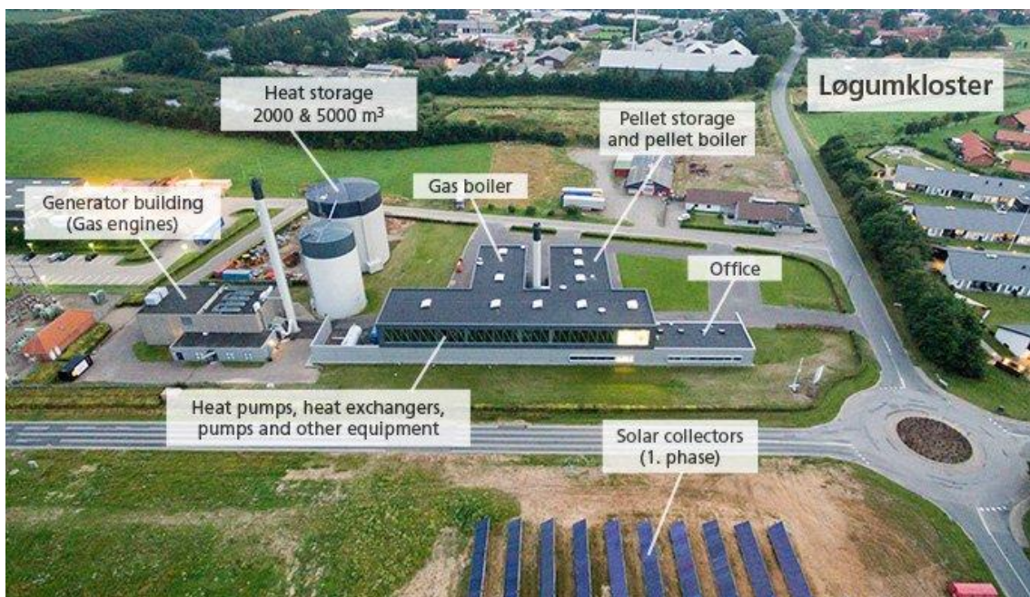
Figure 27. Hybrid district heating plant (CHP) combining wood pellets, solar thermal energy and natural gas in Løgumkloster in Denmark [48].
