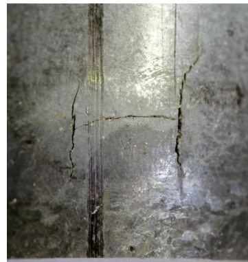
Figure 22: Lower plug welding failure
