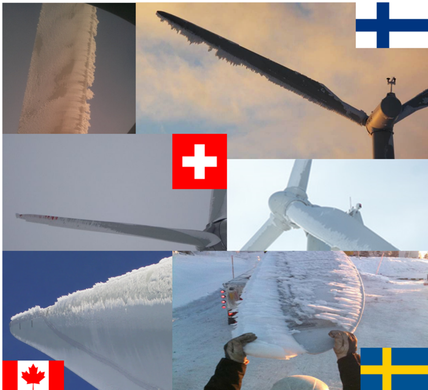
Figure 1. Challenge of ice accretion on wind turbine blades in different countries without blade heating ice protection systems
