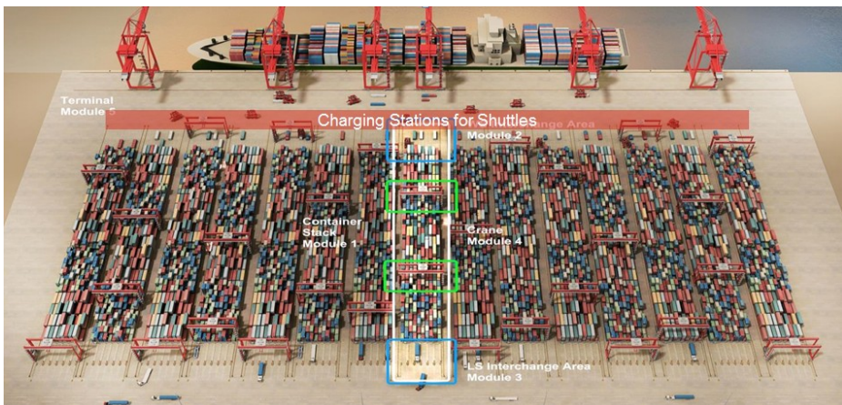
Figure 111. Fast charging stations can be installed along the working route in order to utilise idle time for charging.
