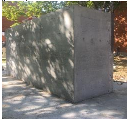
Figure 8. Completed wall mock-up.
