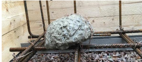
Figure 6. Honeycomb structure prepared in laboratory and sealed with stiff mortar cover to avoid filling of the voids with cement paste from the concrete.
