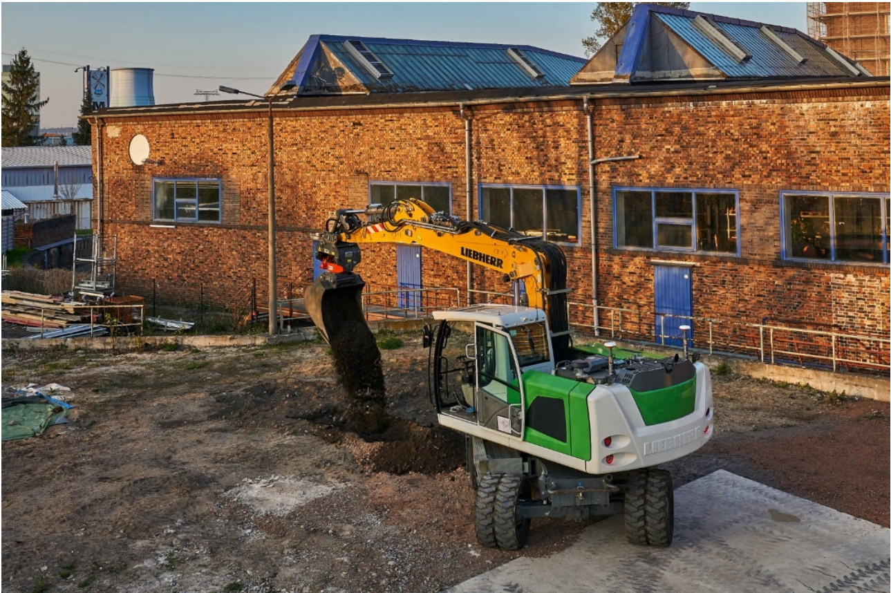
Figure 19. Excavator in operation
