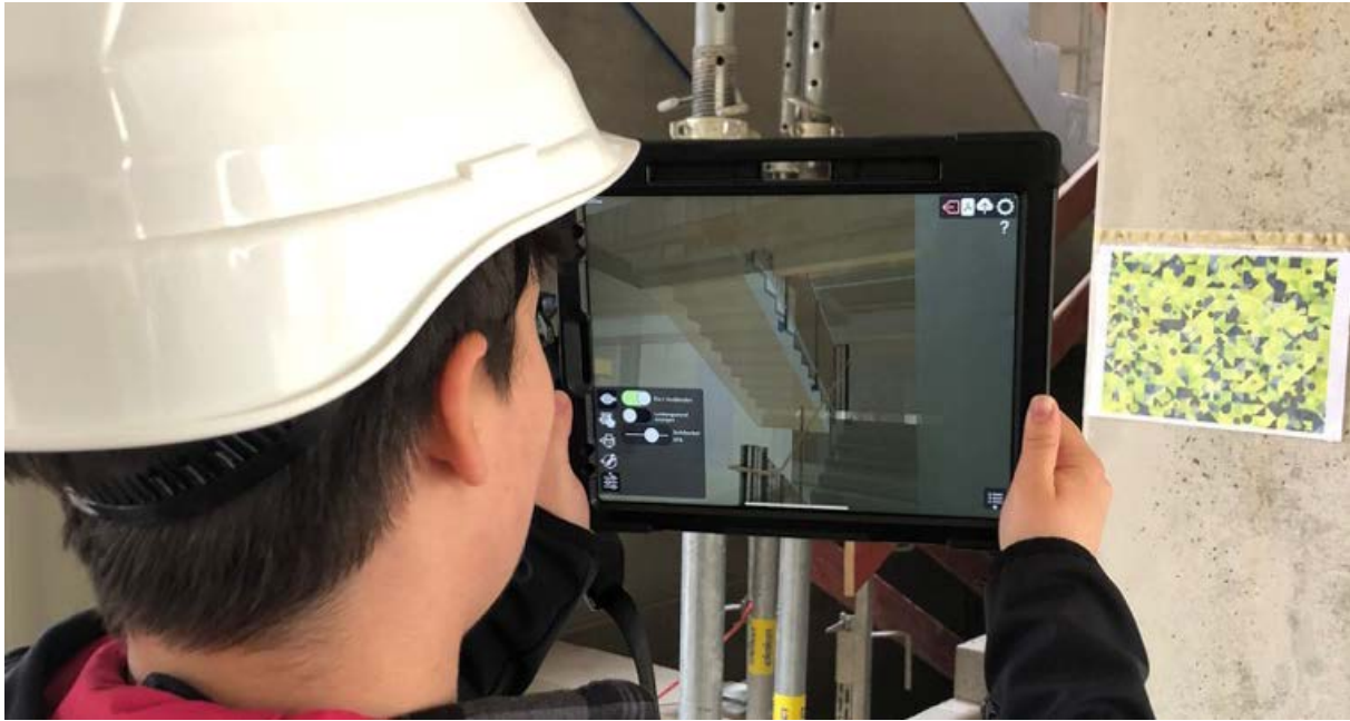
Figure 13. Testing of our prototype on the campus' construction site.
