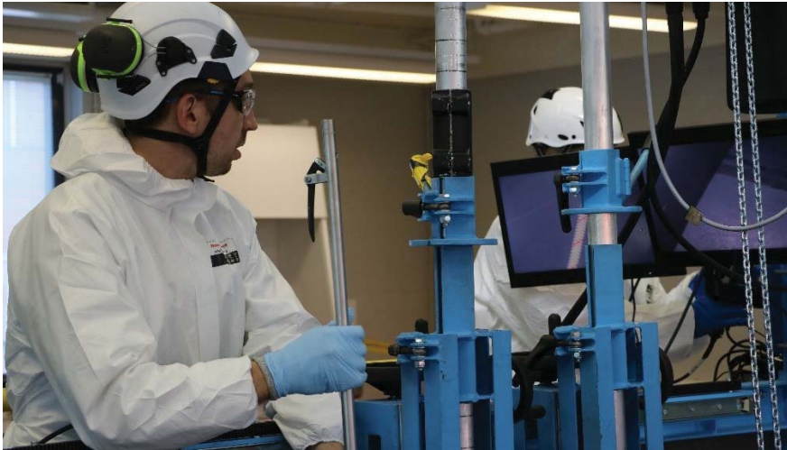
Figure 6. Operator at work during the dismantling of reactor core internals of the FIR 1 research reactor.
