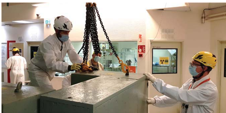
Figure 26. Operators preparing radiation shields for handling dry spent fuel in the FiR 1 reactor hall in 2020.
