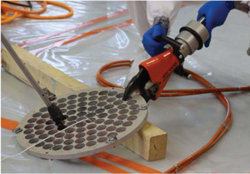
Figure 32. Some of used reactor components are classified as dual-use items (other nuclear material) while they are also forming different types of radioactive waste. During decommissioning, the maintenance of the facility's nuclear materials inventory bookkeeping requires special attention and close communication with the regulator and nuclear safeguards organizations. The core grid plate of the FiR 1 research reactor is another example.
