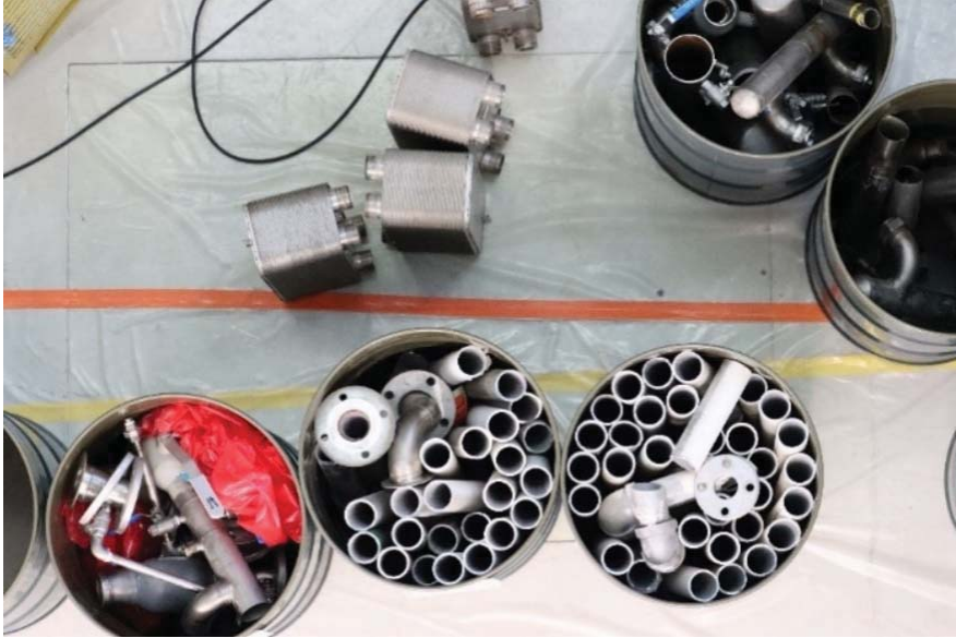
Figure 3. Decommissioned primary circuit tubes for free release from the FIR 1 reactor.
