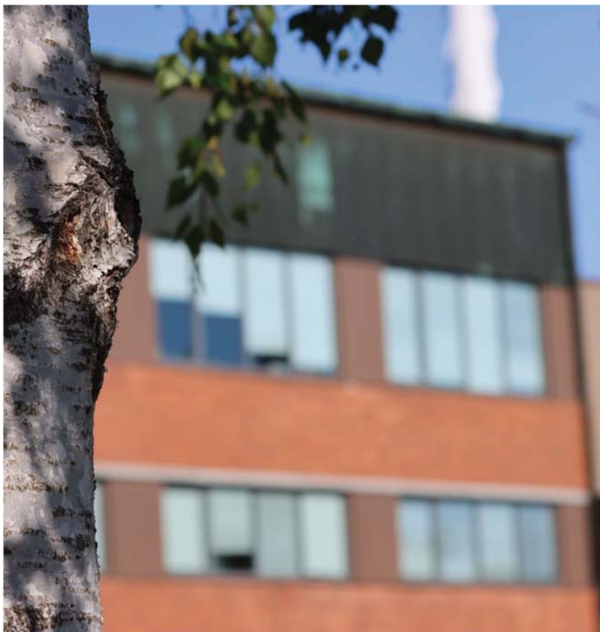
Figure 30. The reactor building looks like a normal office from outside.
