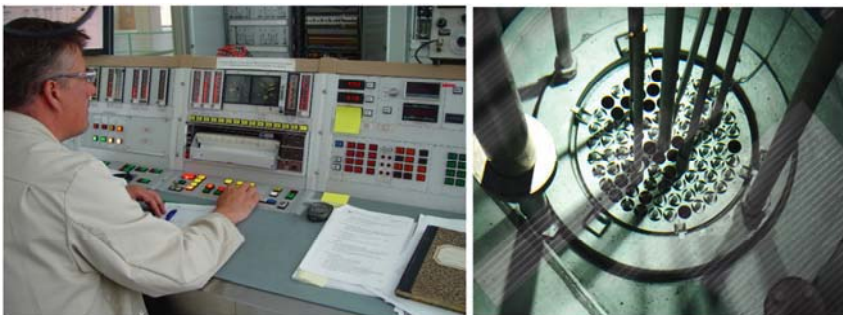
Figure 25. Reactor operator just about to shut down FiR 1 for the last time on 30 June 2015. At the end of the same year, the core was made permanently subcritical by removing enough fuel elements.
