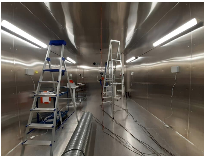
Figure 2. The chamber during installations
