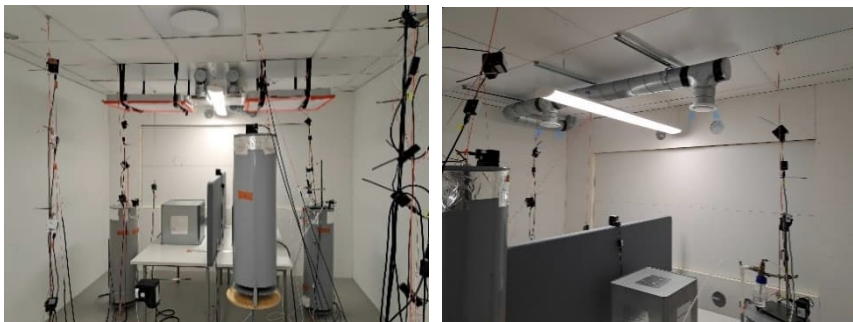
Figure 4. Special ventilation approaches: additional inlets above the workstations (left), and additional exhausts above the workstations combined with displacement ventilation (right).
