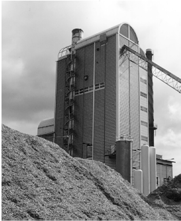
Figure 2. Värnamo biomass IGCC (Sydkraft AB and Foster Wheeler Energia Oy).
