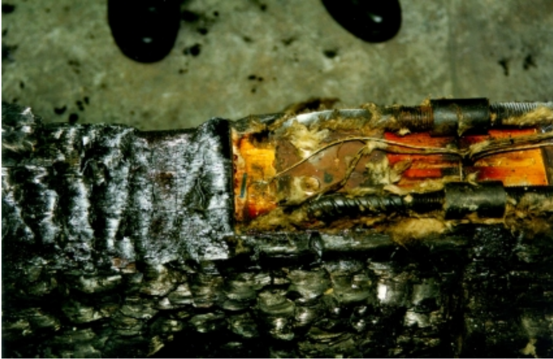
Figure 14. The connection of Beam 1 after removal of the fire protection.
