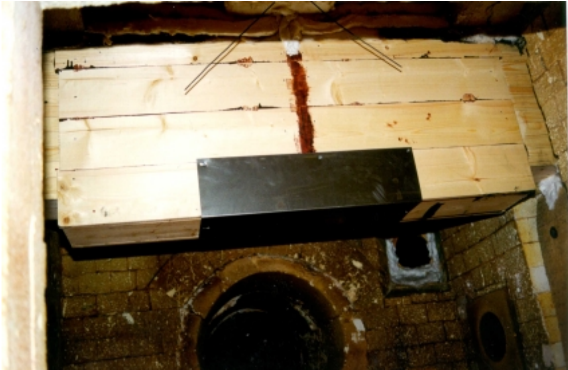
Figure 6. Beam 3 prior the test (18.12.1998).
