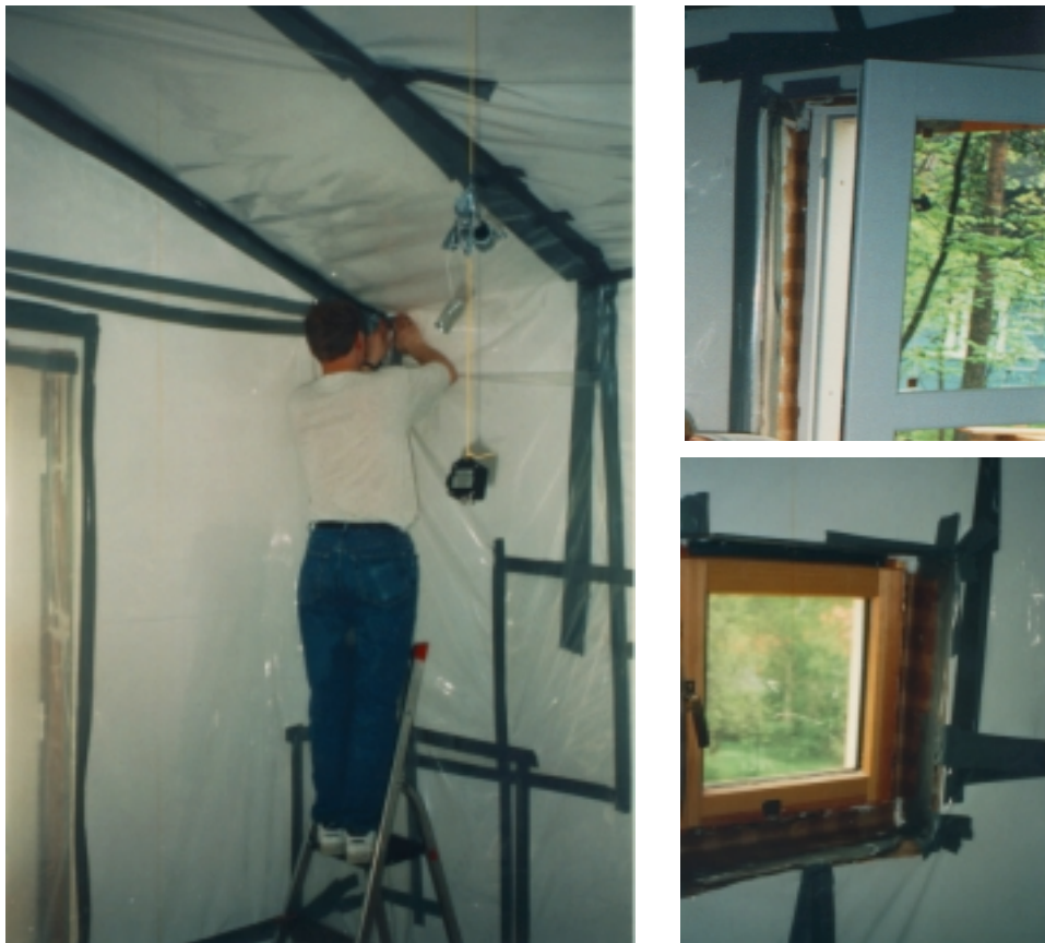
Figure 17. Sealing the test room with polyethylene plastic.
