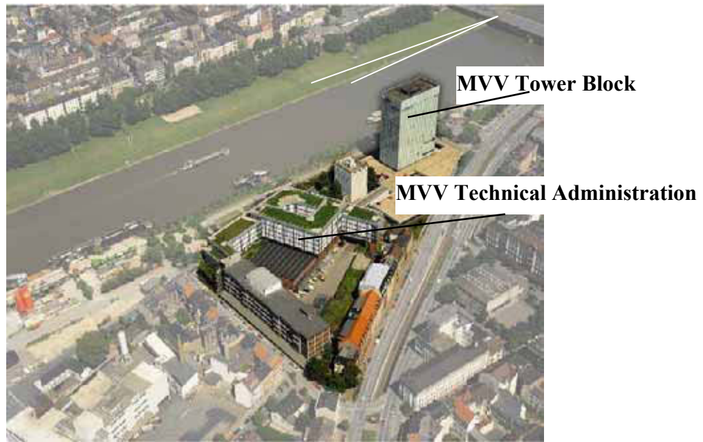
Figure 23. MVV administration building.
