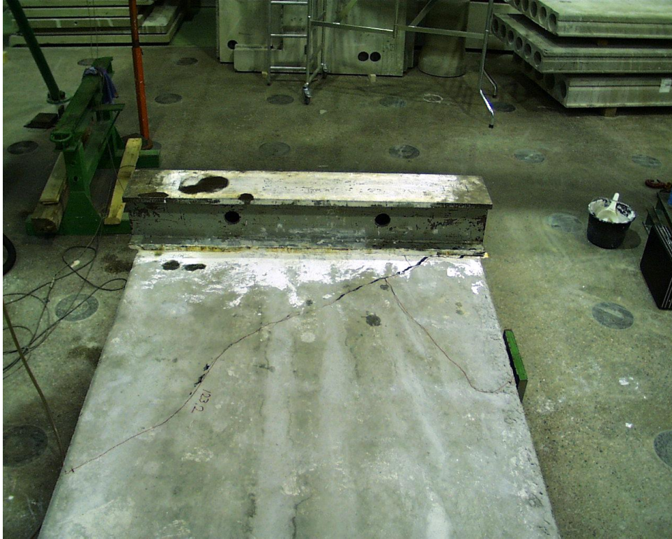
Fig. 13. PT200A. Cracks on the top of the slab after failure.
