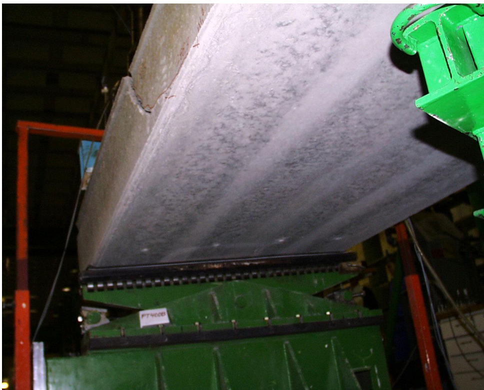
Fig. 36. PT400B. Soffit of slab after failure.
