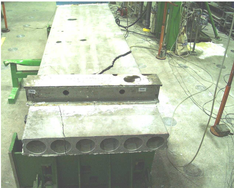
Fig. 14. PT200A. Cracking pattern at the cantilevered passive end after failure.
