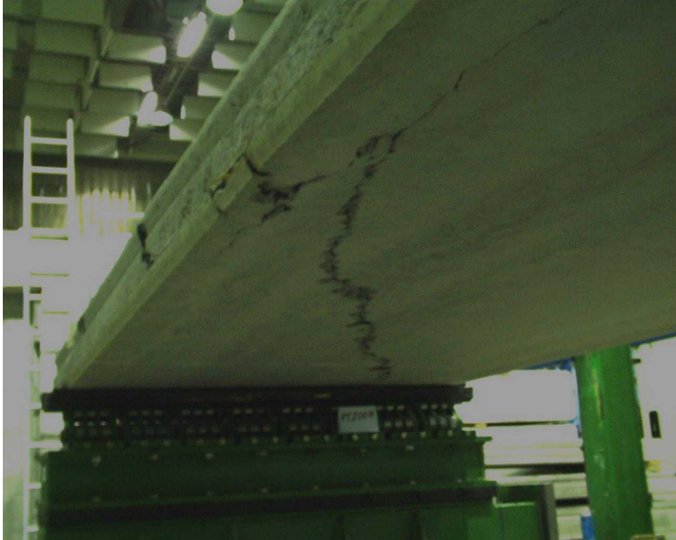
Fig. 21. PT200B. Cracking pattern after failure.
