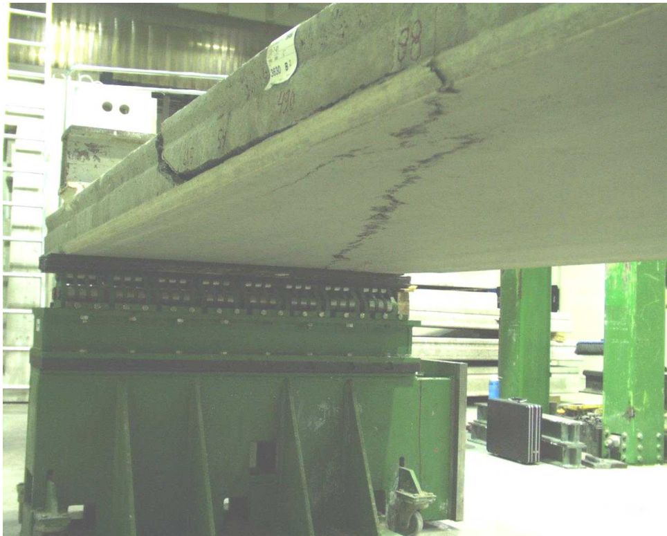
Fig. 16. PT200A. Cracking pattern at the soffit of the slab after failure.
