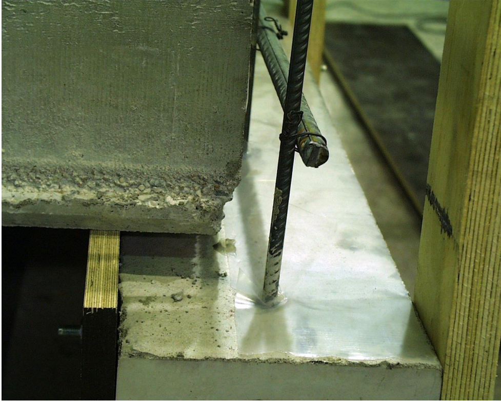
Fig. 5. Top surface of beam before grouting. Note the plastic sheet.
