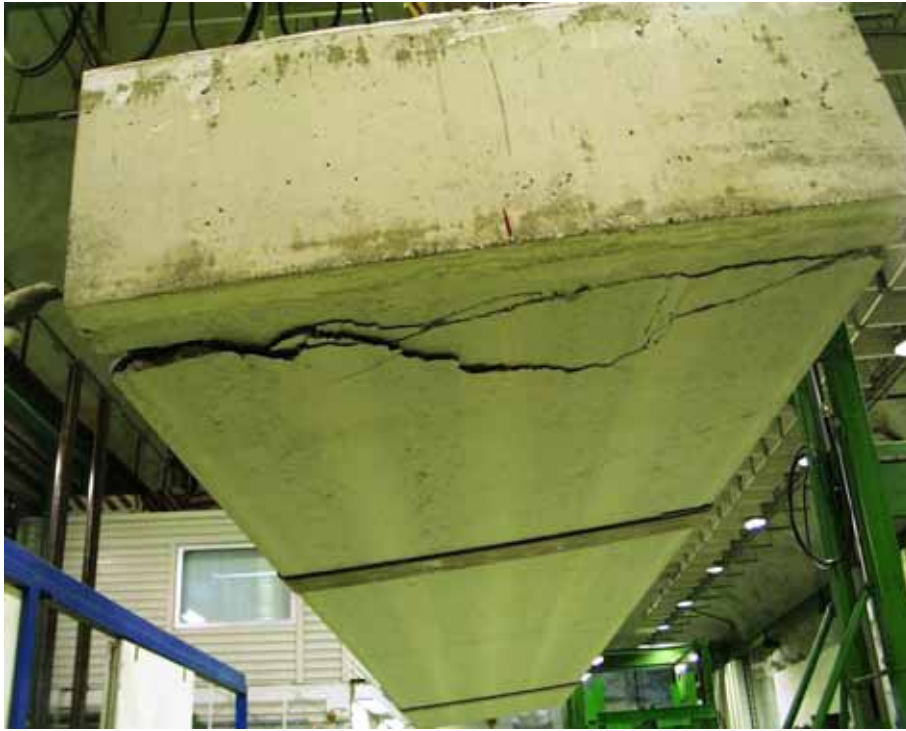
Fig. 55. ST400G1, active end, soffit after failure.
