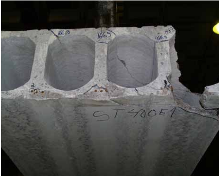
Fig. 21. ST400E1. Soffit after failure.
