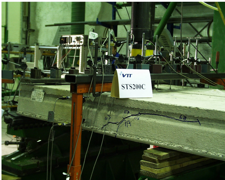
Fig. 26. STS200C. Cracking pattern after failure. Northern edge.
