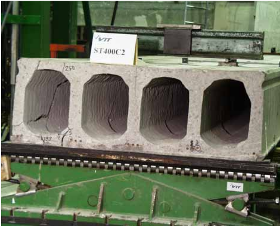
Fig. 11. ST400C2. Cracks in webs after failure.
