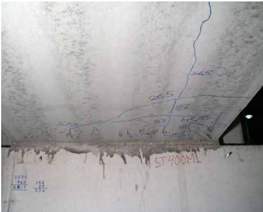
Fig. 42. ST400E1M. Cracking of soffit after unloading.
