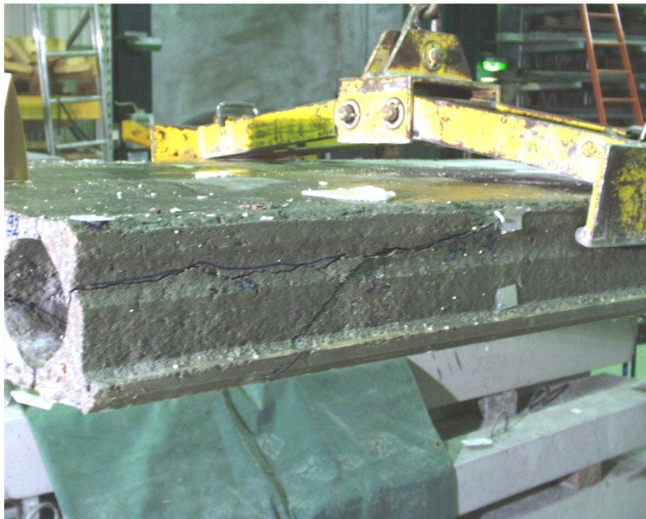
Fig. 16. ST200E1b. Northern edge after failure.
