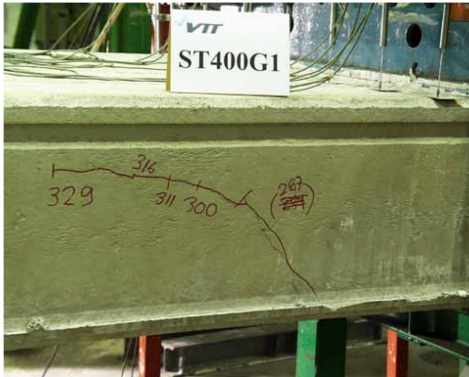
Fig. 51. ST400G1, North edge, cracks before failure.
