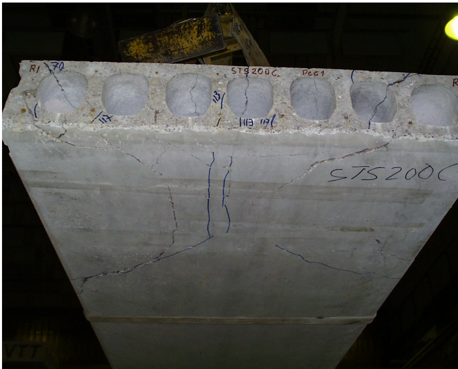
Fig. 30. STS200C. Soffit after failure.
