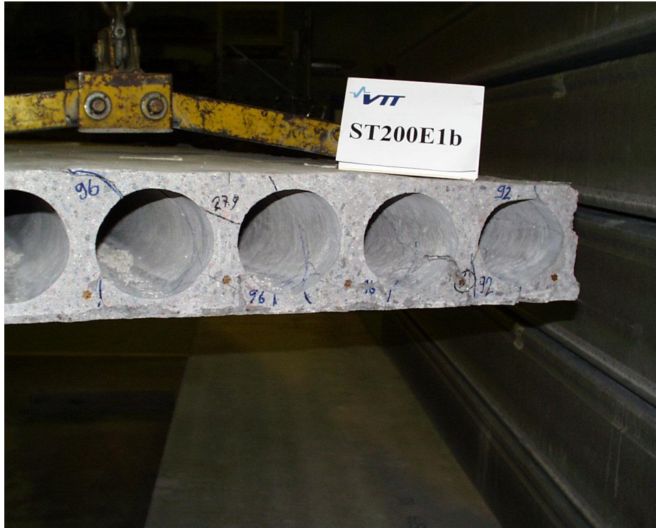
Fig. 19. ST200E1b. Cracking pattern in webs.
