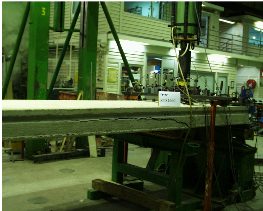
Fig. 28. STS200C. Cracking pattern after failure. Southern edge.
