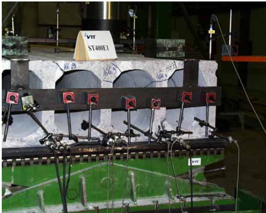
Fig. 16. ST400E1. Cracks at the end after failure.
