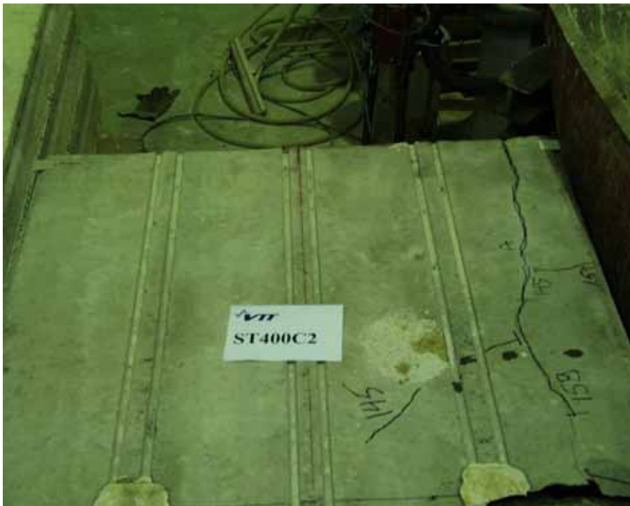
Fig. 14. ST400C2. Top surface after failure. A thin crack until letter A was observed before loading.
