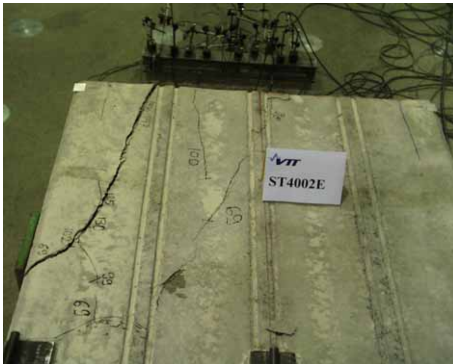
Fig. 26. ST4002E. Top surface after failure. Note the thin crack at the upper right corner of the figure. This crack existed before loading.
