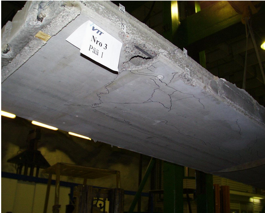
Fig. 41. FT200:12. End 1 of slab 3 after demolishing of floor.
