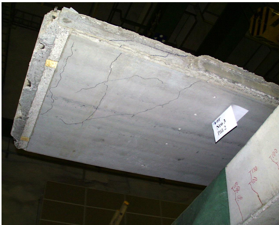
Fig. 42. FT200:11. End 2 of slab 3 after demolishing of floor.
