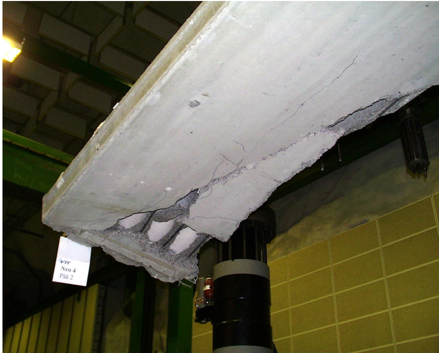
Fig. 37. FT200:11. End 2 of slab 4 after demolishing of floor.
