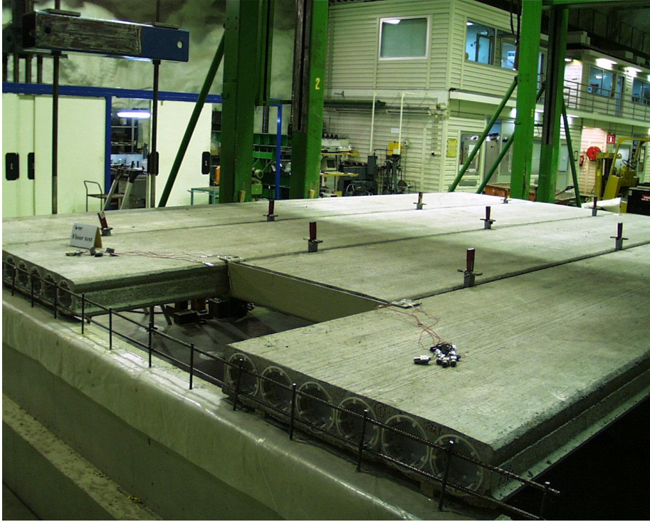
Fig. 7. Overview on floor before grouting.
