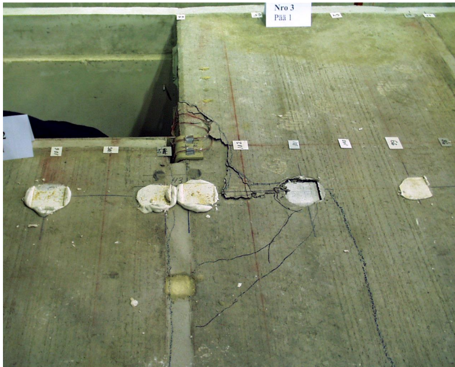
Fig. 25. FT200:12. Cracks on top surface of slab 3 after failure.
