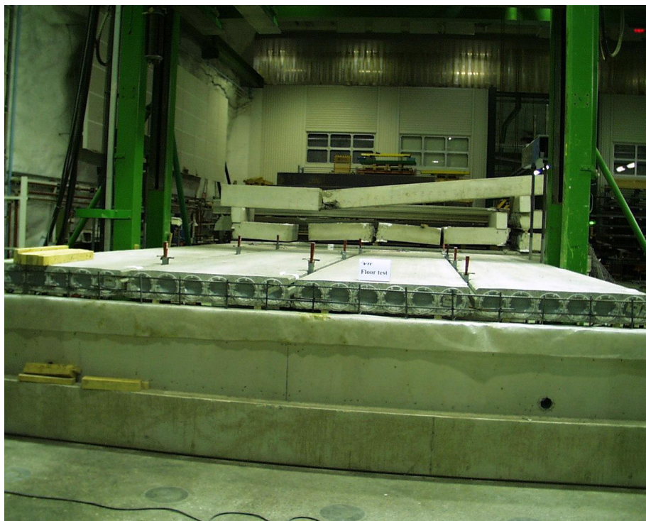
Fig. 6. Overview on floor before grouting. The vertical objects in the joints are wedges.
