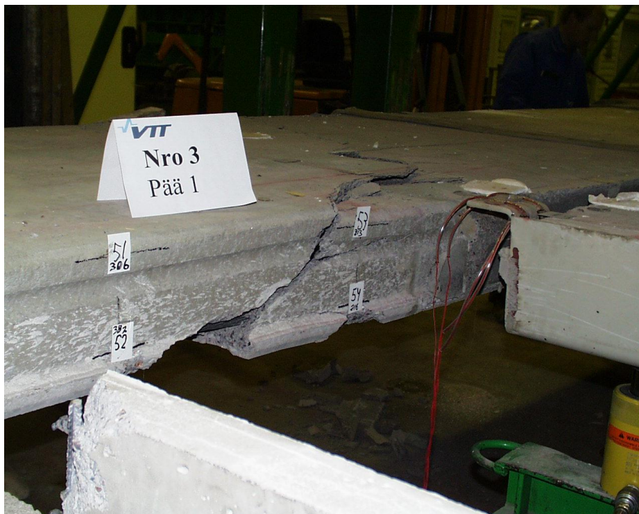
Fig. 40. FT200:12. End 1 of slab 3 during removal of slab 2.
