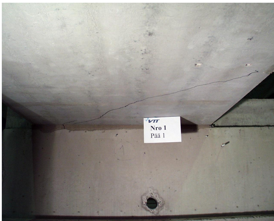
Fig. 29. FT200:12. Cracks on soffit of slab 1 after failure.
