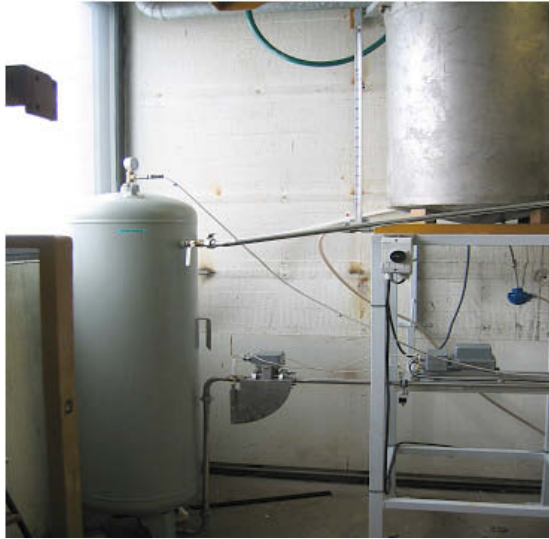
Figure 5.31. The pressurized feed tank on the left (D101) with a tube coming from the bottom of the tank leading to ball valve (VO1). On the left upper corner is the mixing tank (D102).
