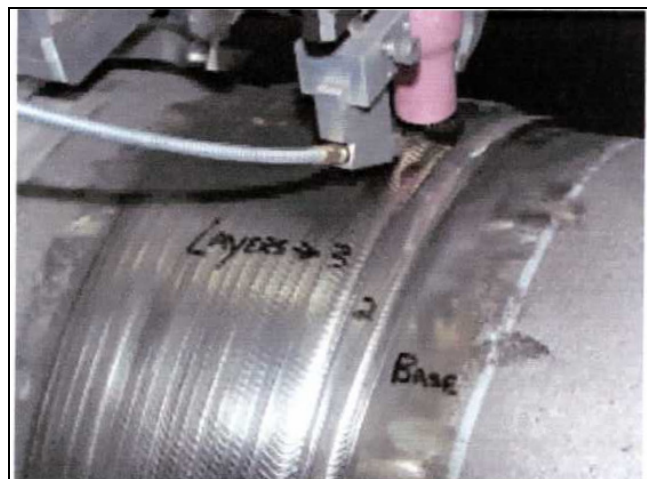
Figure 48. Inconel 52MS structural weld overlay (Findlan et al. 2005).
