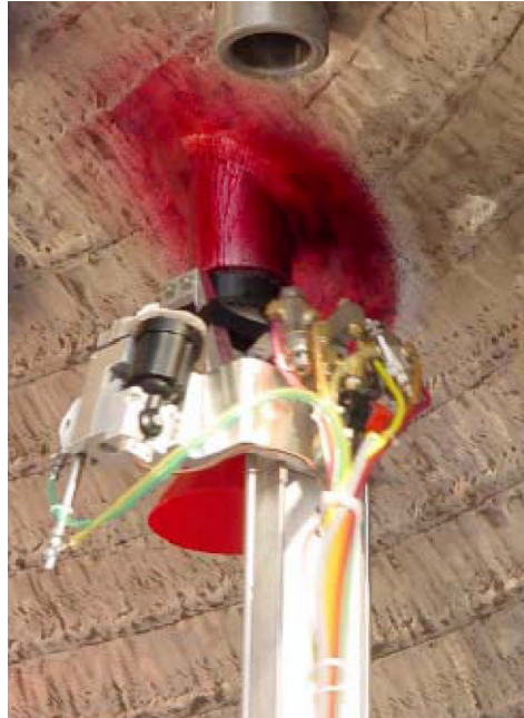
Figure 113. Dye penetrant testing of the vessel head penetration (Lareau 2005a).
