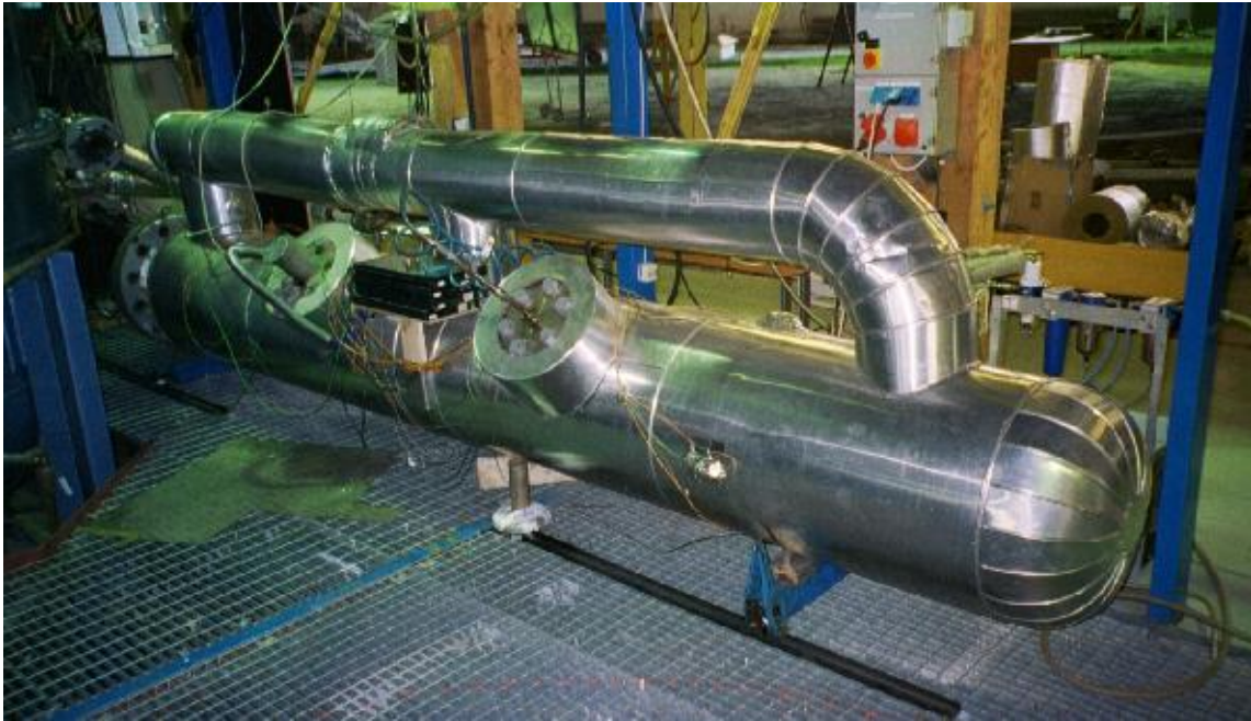
Figure 126. The test section of the Horizon facility (originally one of the steam generators from the PACTEL facility).
