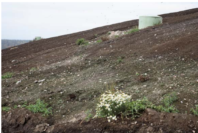
Figure 24. Landfill gas wells at a freshly covered landfill area.
