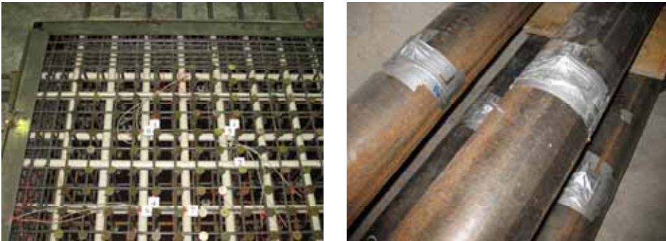
Figure 5. Strain gauges fixed on reinforcement (left) and on back pipes (right).
