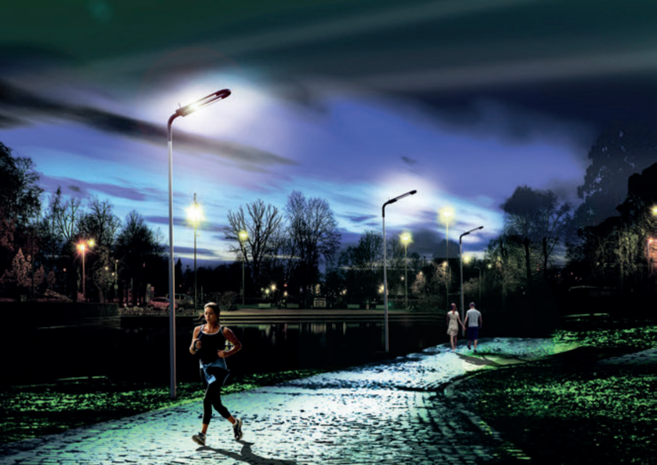
FIGURE 4.10. Intelligent LED streetlights for energy saving. The lights are equipped with sensors to detect people and ambient light conditions. They also communicate with each other, adjusting light levels optimally for the street. (Picture: AthLEDics project.)
