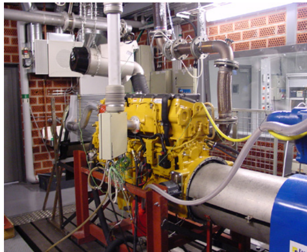
VTT has several dynamometers for engine-only research and development.
