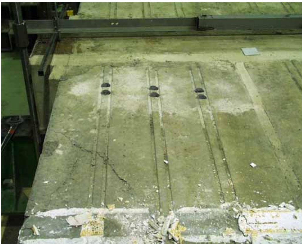
Fig. 20. Failure pattern on the top of slab 1 after removing the loading equipment and drilling the cores.
