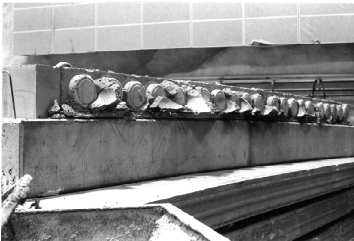
Fig. 13. The middle beam after the loading test, on the edge of the slab units no 5 - 8.
