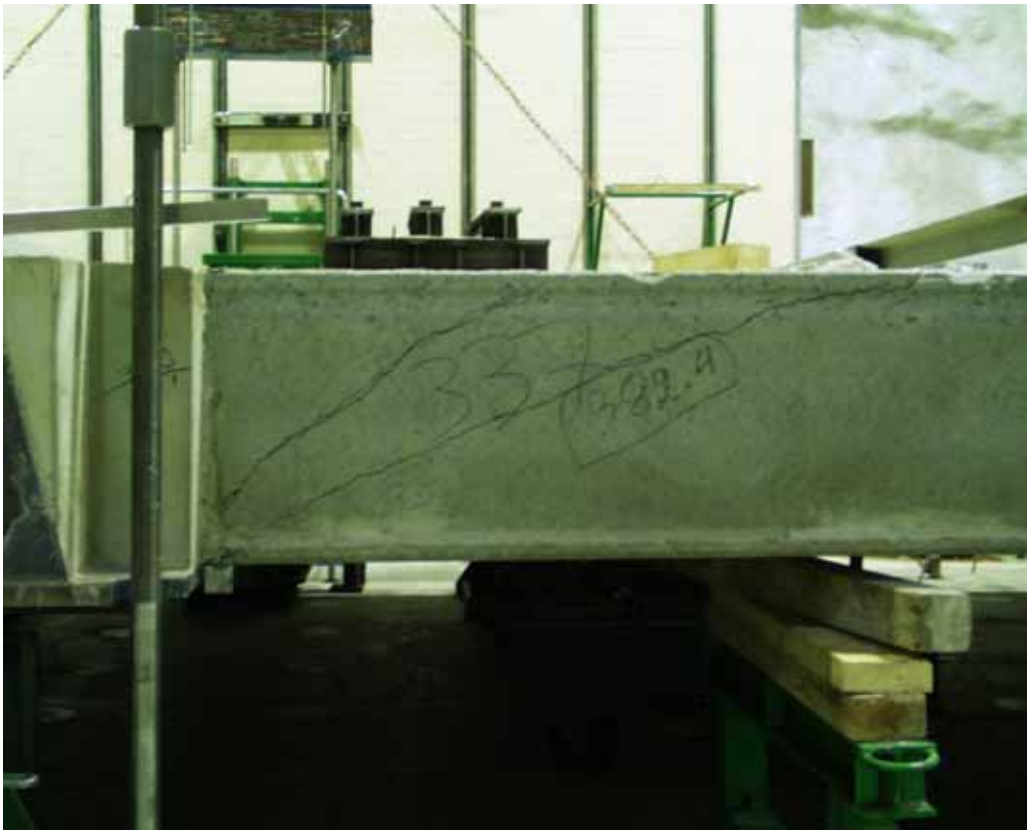
Fig. 19. Shear cracks in slab 1 after removing the loading equipment.
