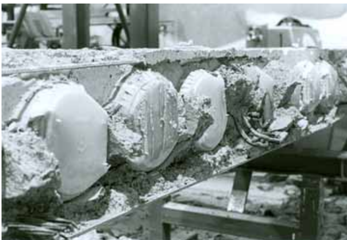
Fig. 17. Detail of middle beam after removing slab units.
