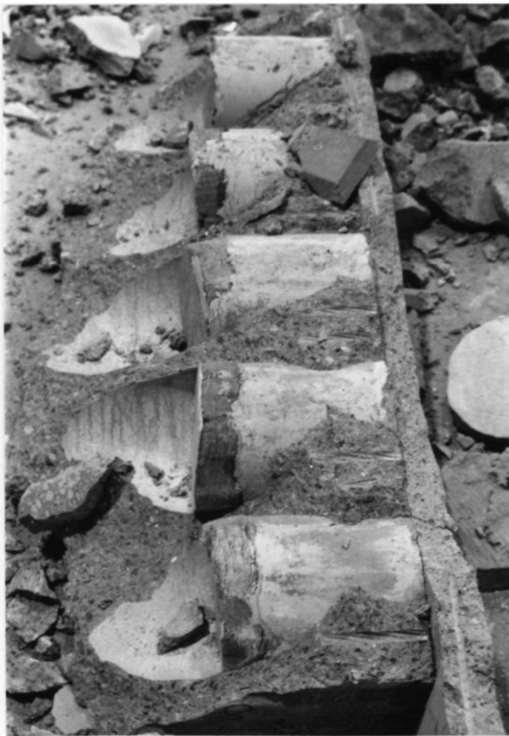
Fig. 19. Void filling at end of slab unit no 8 (upside down).
