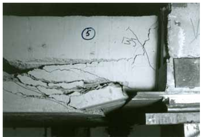
Fig. 6. Detail of slab unit 5 after failure.
