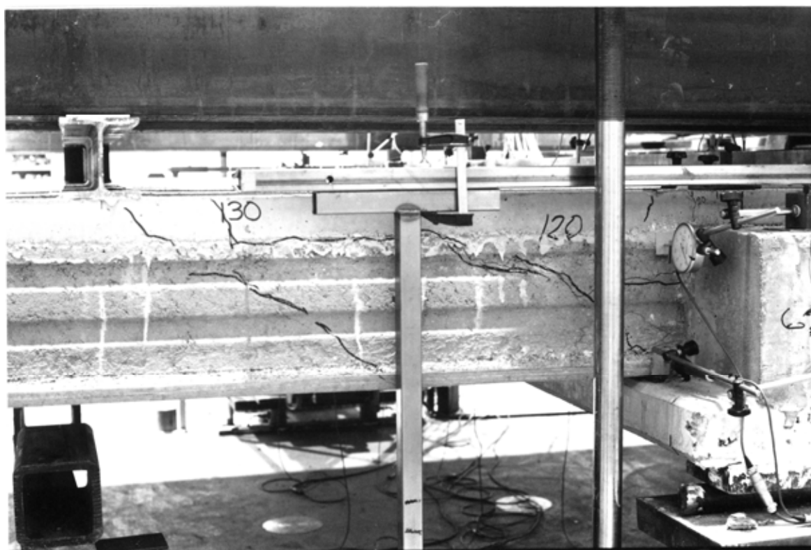
Fig. 12. The cracks in the longitudinal edge of the slab unit no 4, near the middle beam, at failure.
