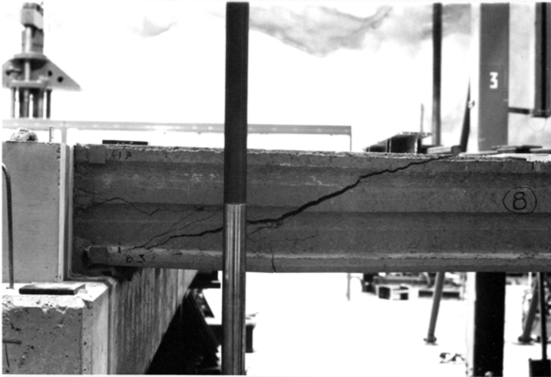
Fig. 9. The cracks in the longitudinal edge of the slab unit no 8, near the middle beam, at failure.
