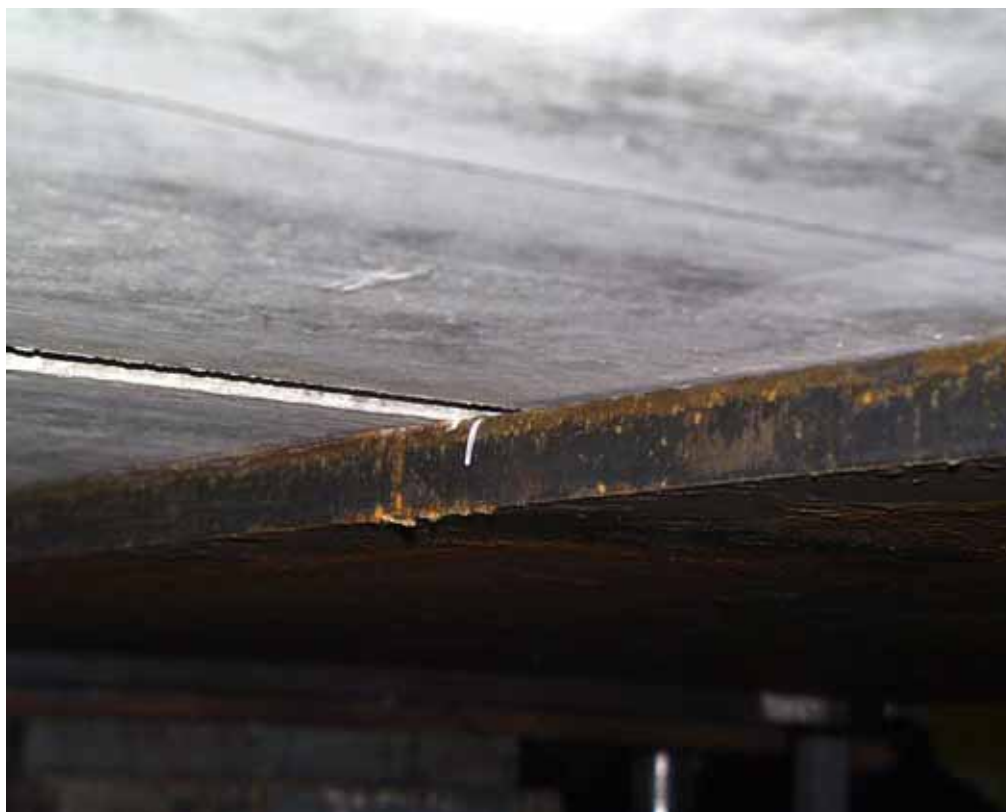
Fig. 13. Bottom flange of middle beam supporting slabs.
