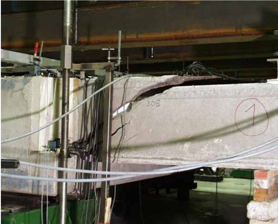
Fig. 17. Failure in slab 1. Photographed after stage II. In stage I, the failure crack was the same but much thinner.
