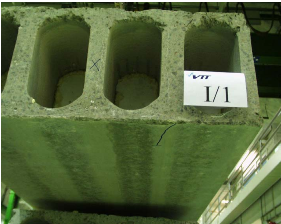
Fig. 2. Initial crack in slab 1.
