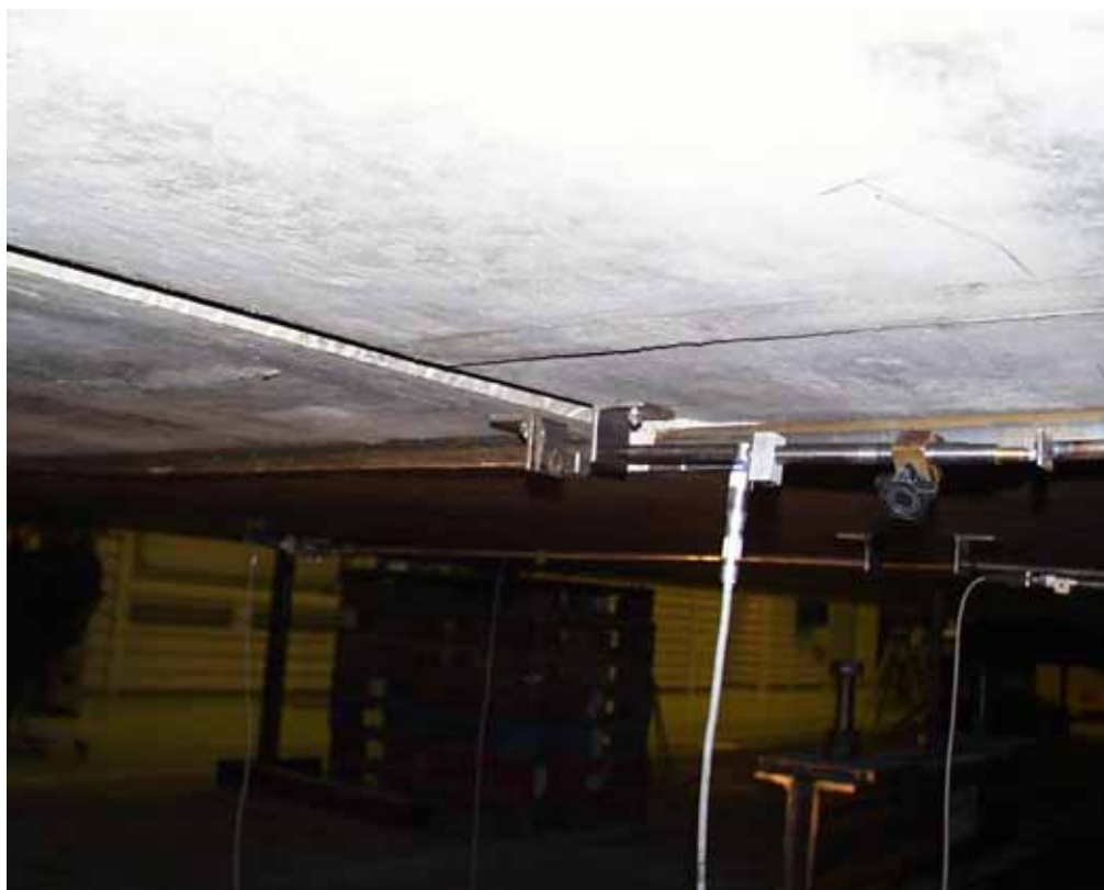
Fig. 14. Equipment for measuring average transverse strain of the soffit.
