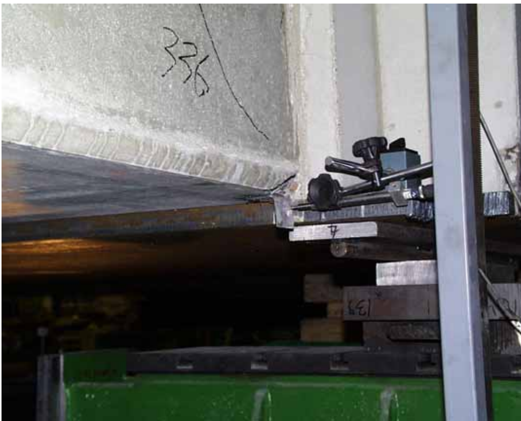
Fig. 12. Transducer, fixed to the bottom flange of the middle beam, measuring sliding of slab along beam.
