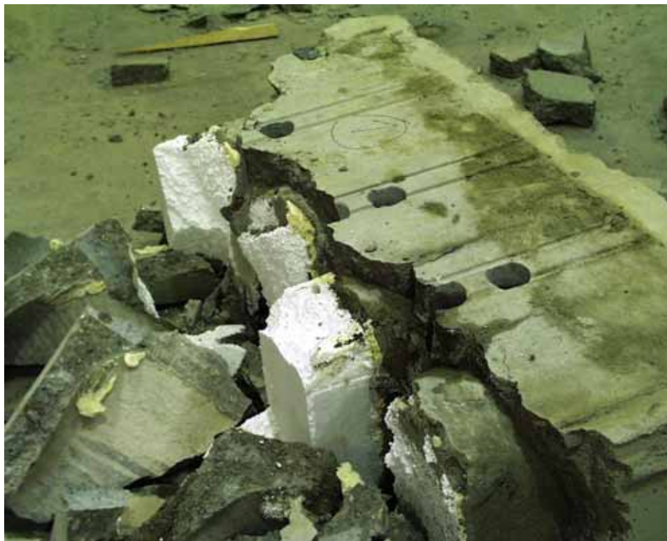
Fig. 23. Core filling in slab 1.
