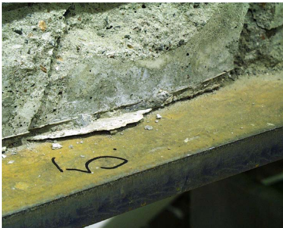
Fig. 58. Grout below slab 5.
