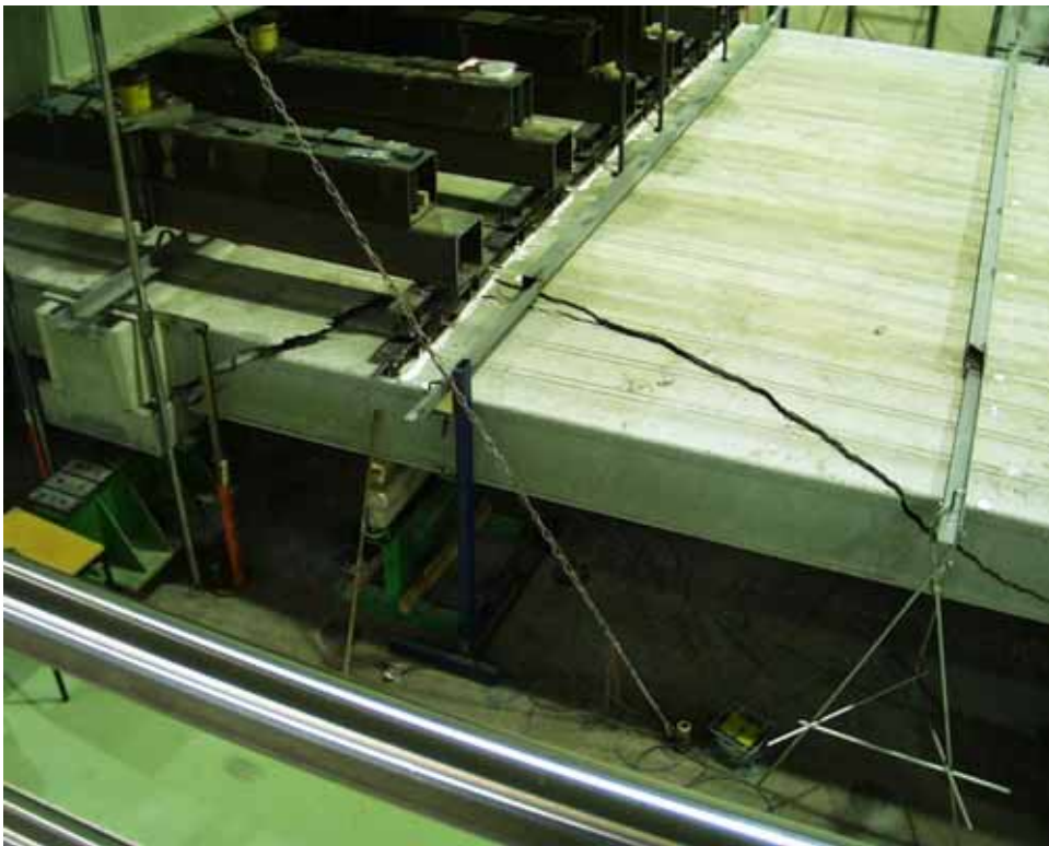
Fig. 18. Failure mode in slab 1.
