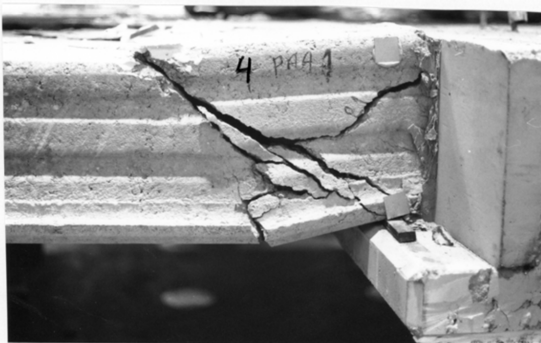
Fig. 10. Failure of slab unit no 4.
