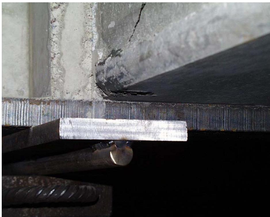
Fig. 41. Slab 1 after test.
