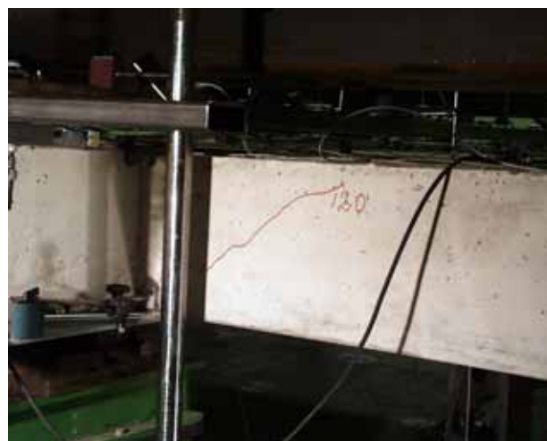
Fig. 10. Diagonal crack in slab 8 after failure.
