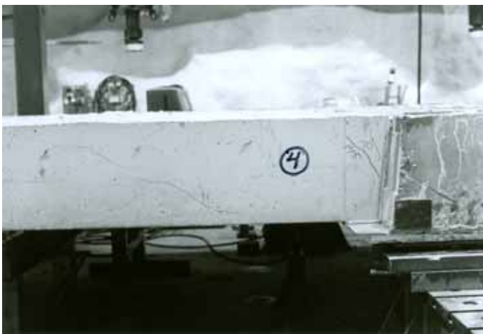
Fig. 11. Cracking pattern of slab unit 4 after failure of slab units 5–8.
