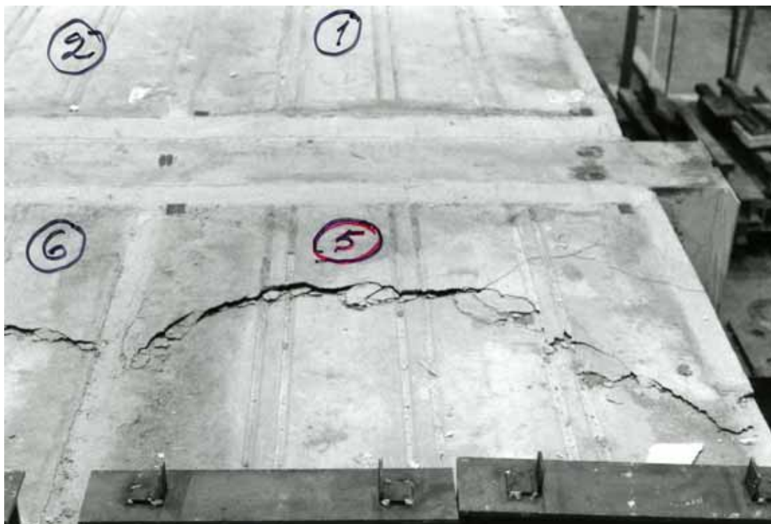
Fig. 18. Top surface of slab unit 5 after failure.
