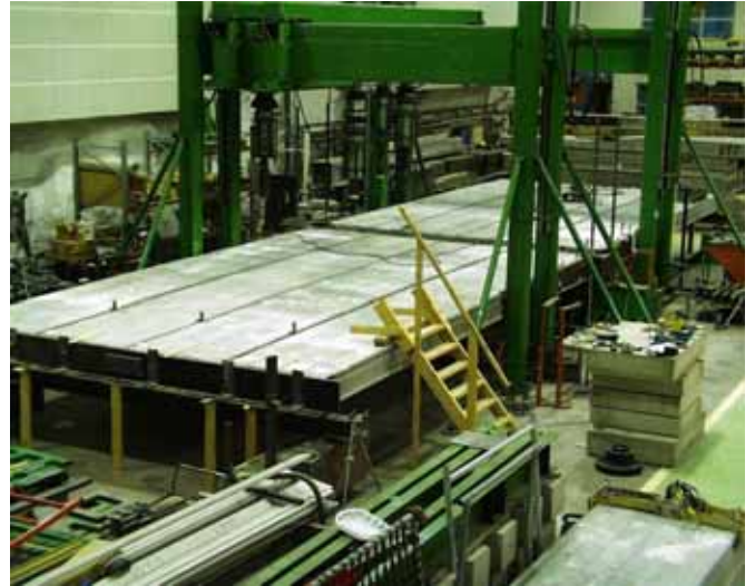
Fig. 8. Test floor before grouting. Note the wedges in the joints to facilitate the demolishing of the floor after the test. To eliminate the contact between the floor and the loading frame, the outermost webs of the slabs were made thinner at the legs of the frame.
