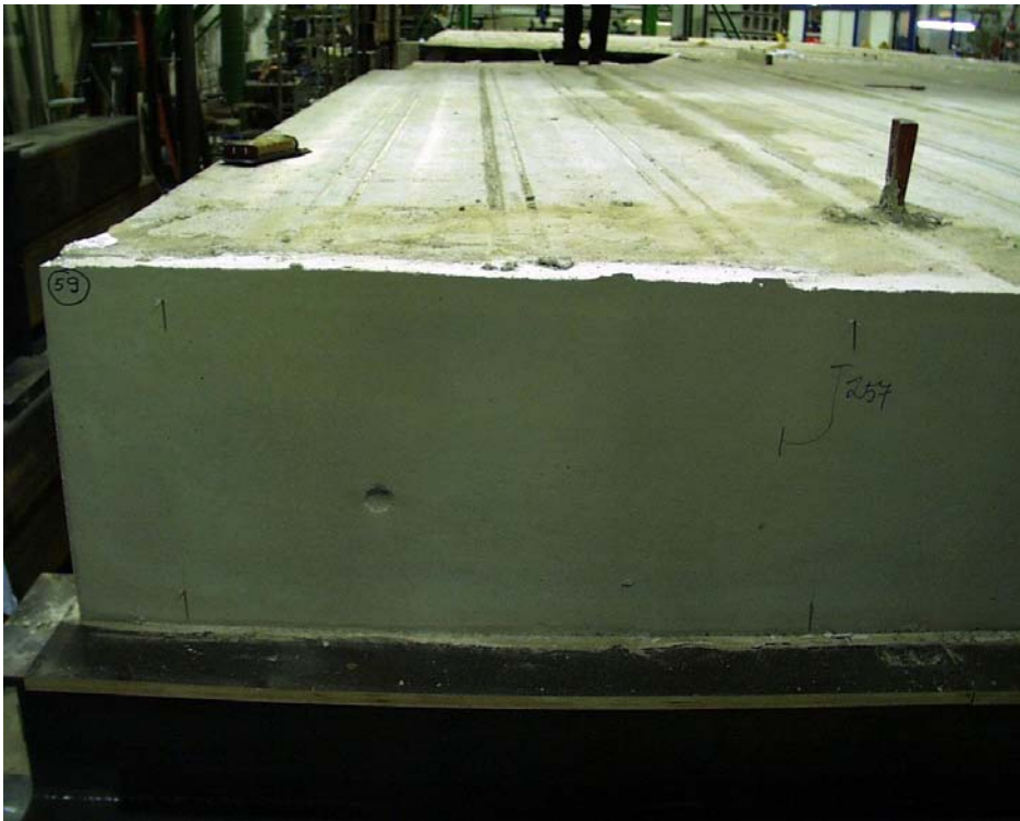
Fig. 39. Slab 12 after test. Cracks in tie beam.
