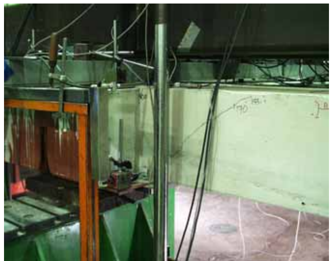
Fig. 24. Cracks in slab 1 after failure.
