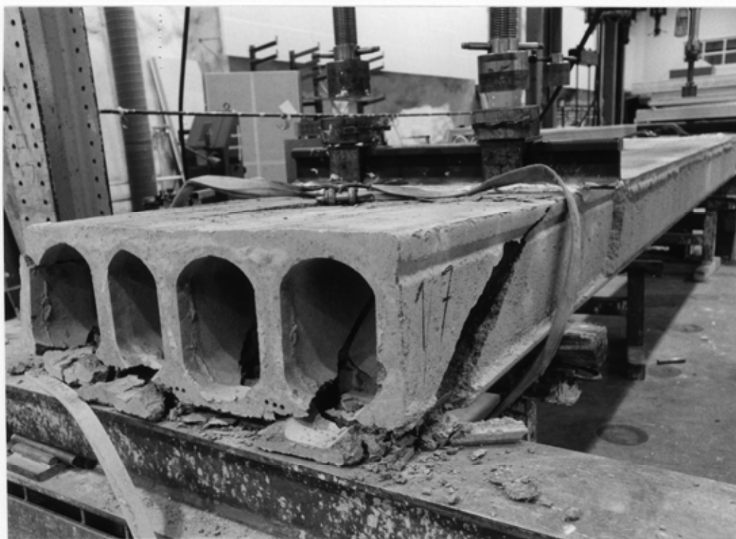
Fig. 17. Failure pattern of slab unit no 7 in reference test.
