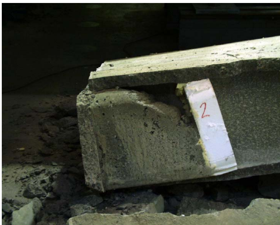
Fig. 50. Concrete filling in one core of slab 2. Note that the polystyrene plug is inclined due to the casting pressure. Consequently, the length of the filling at the bottom is greater than 400 mm.
