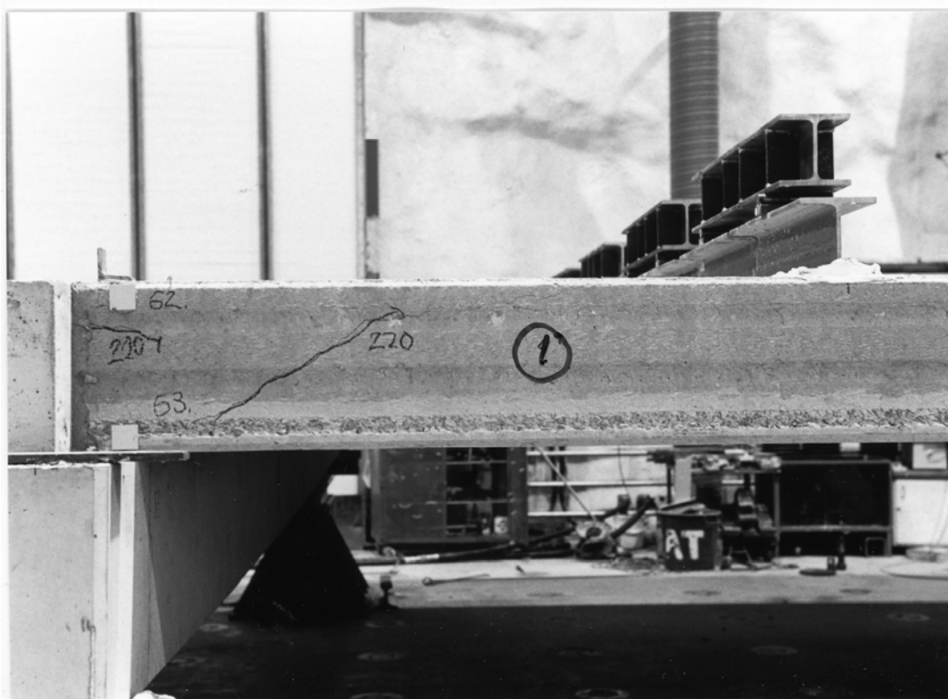
Fig. 10. Cracking pattern of slab unit No. 1 after failure of slab unit No. 7.
