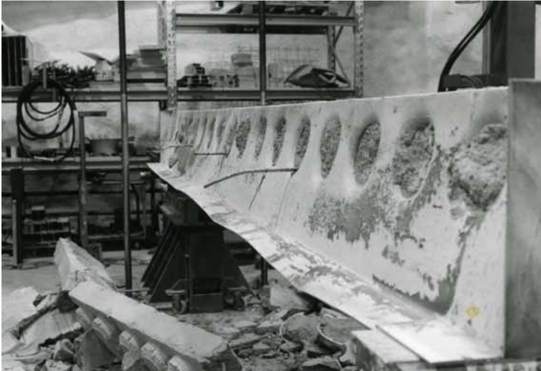
Fig. 27. Web and deformed ledge of middle beam after removal of slab units and joint concrete. The tie bars penetrating the beam have been flame-cut after the test.
