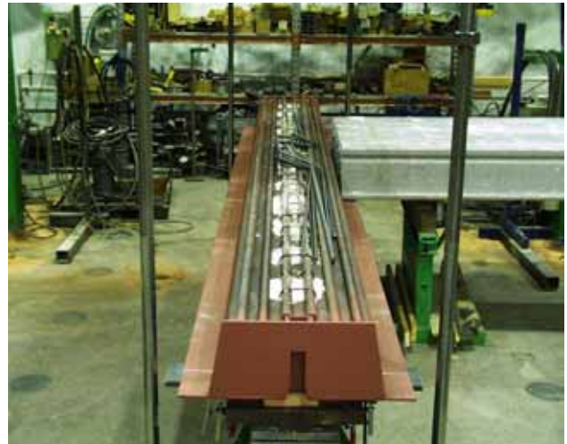
Fig. 2. A-beam. Suspension bars temporarily stored on the top of the beam.
