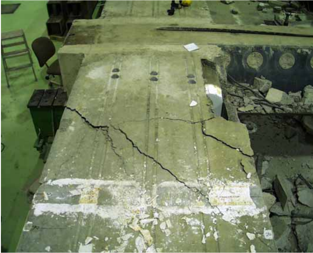
Fig. 21. Slab 1 after removing slabs 2–6 and 8–12.
