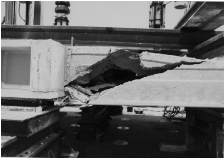
Fig. 15. Failure of slab 8.
