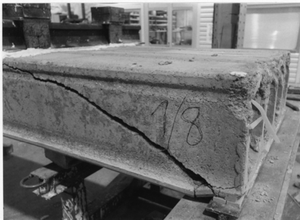
Fig. 18. Failure pattern of slab unit no 8 in reference test.
