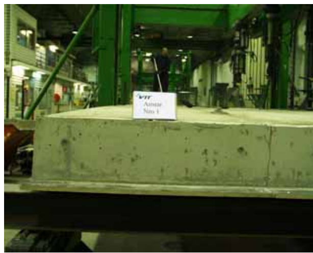
Fig. 28. Cracks in Western tie beam after failure. Slabs 1 and 2.
