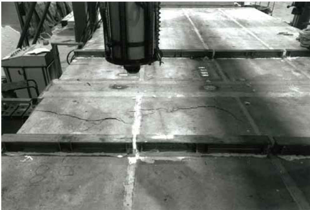
Fig. 18. Top surface of slabs 1 (on the left), 2 and 3 after failure.
