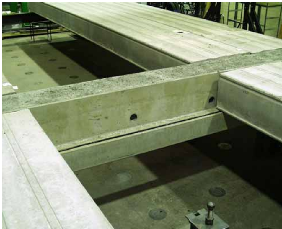
Fig. 3. Installing slabs on PC beam.
