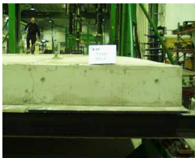
Fig. 30. Cracks in Western tie beam after failure. Slabs 3 and 4. The red colour and letter A refer to an initial crack.
