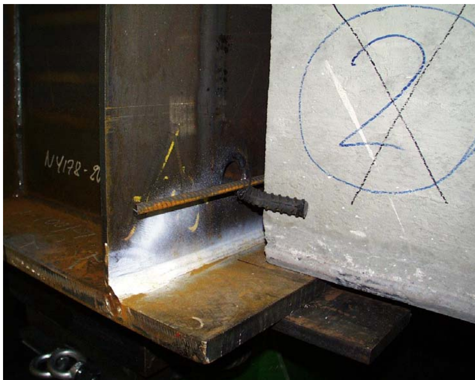
Fig. 13. A short, bent tie bar, outer edge of slab 1.
