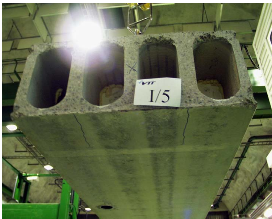
Fig. 6. Initial cracks in slab 5.
