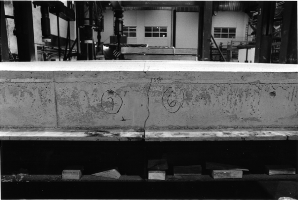
Fig. 9. A crack in the middle of the concrete tie beam, between the slab units no 6 and 7.
