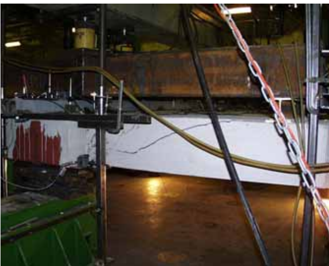
Fig. 23. P_{a2} = 155 kN. Wide cracks in slab 8.
