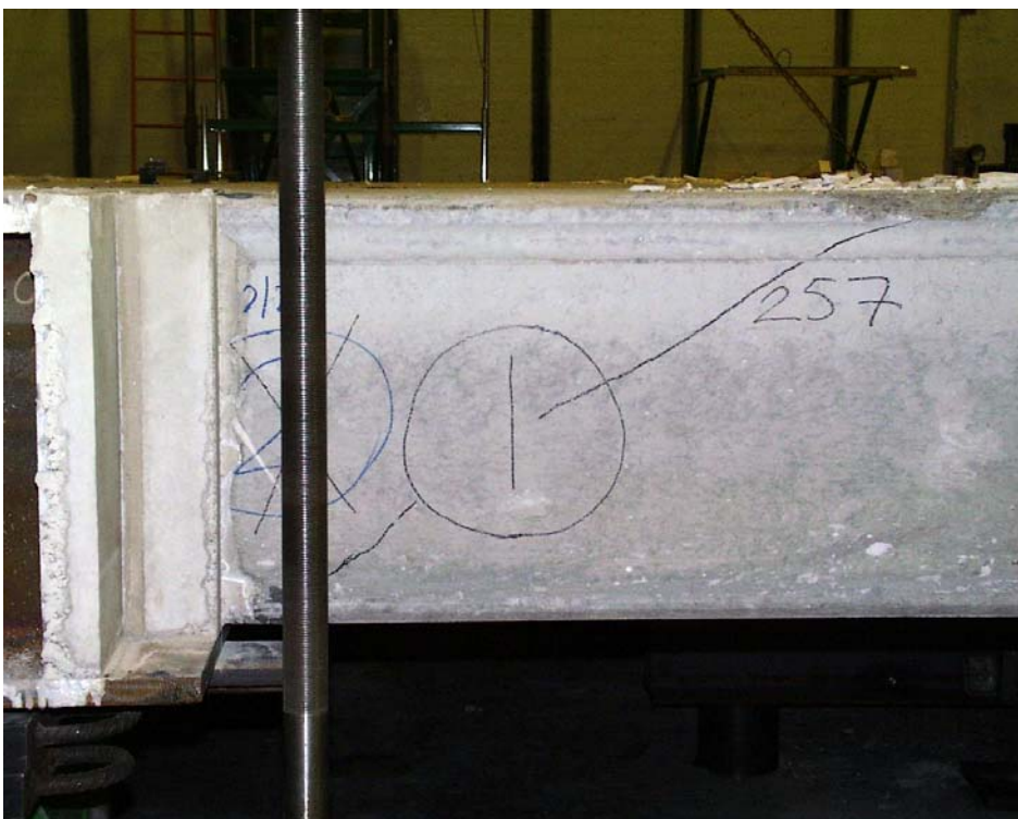
Fig. 40. Slab 1 after test.
