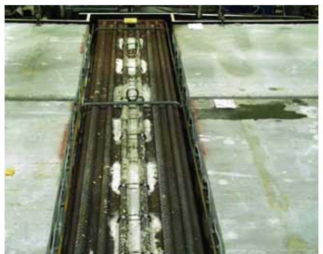
Fig. 6. Middle beam before grouting of joints.
