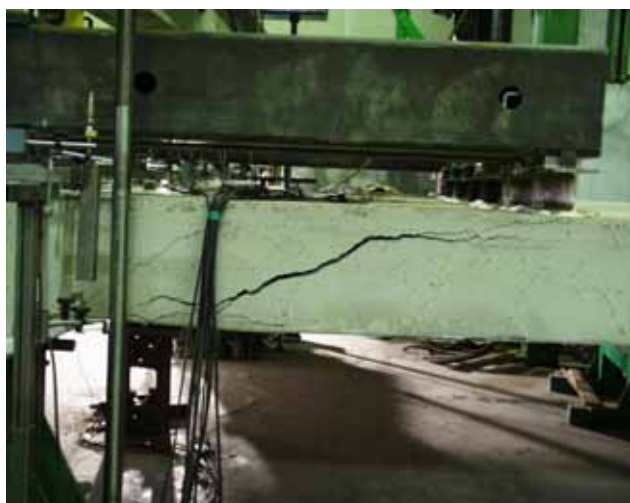
Fig. 9. Failure of slab 1.
