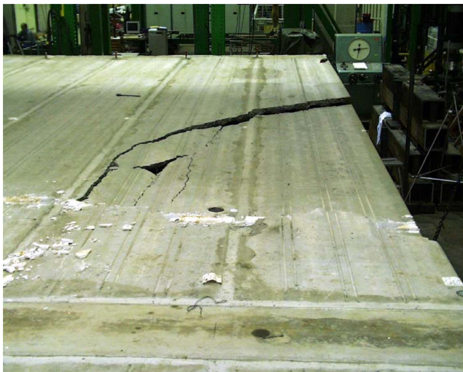
Fig. 33. Slabs 11 and 12 after removing the loading equipment.
