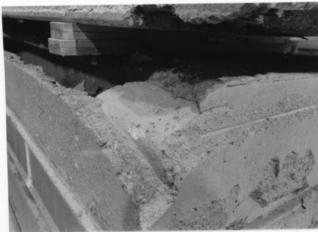
Fig. 9. Filling of outermost hollow core. Note the perfect filling on the top.
