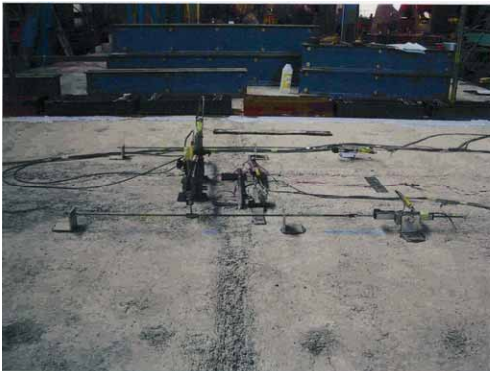
Fig. 2. Equipment for measuring average strain in hollow core slab.
