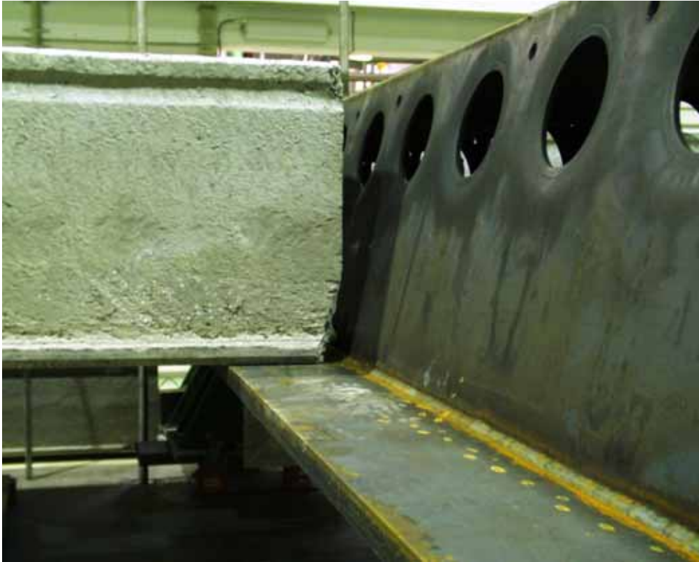
Fig. 3. Slab placed on Delta beam.
