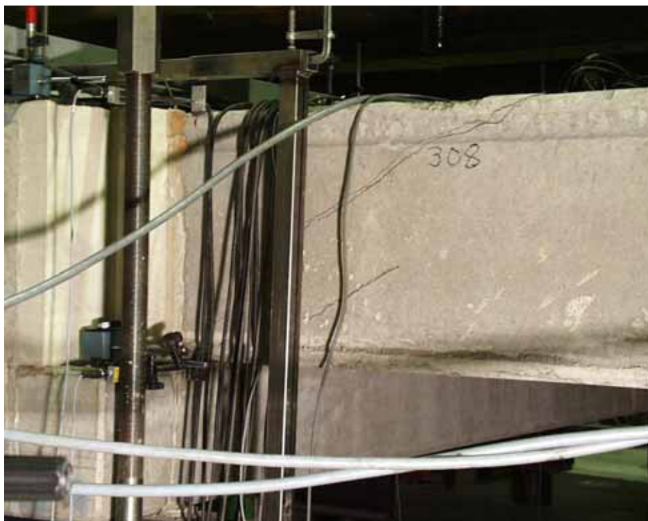
Fig. 15. Shear crack at P_a = 308 kN. The black line drawn 200 mm below the shear crack is a misprint which does not refer to a crack.
