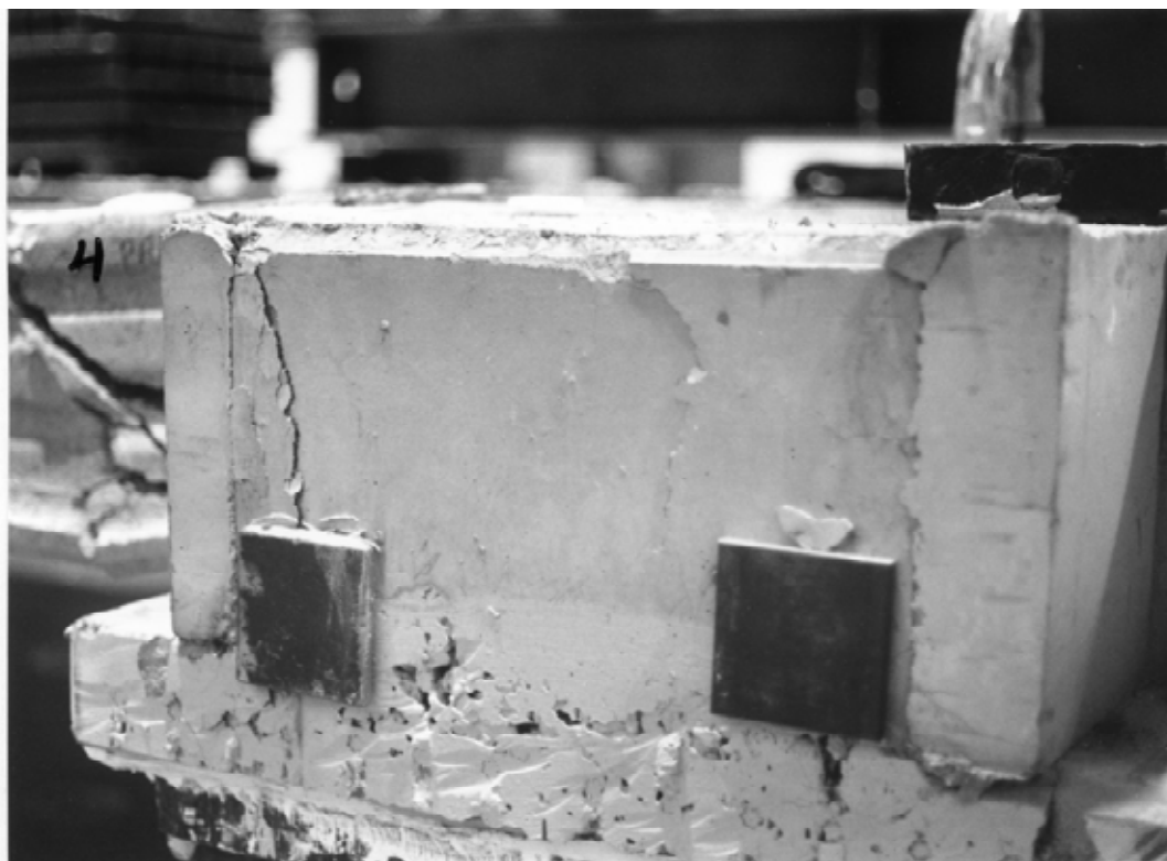
Fig. 22. Cracking of end 2 of middle beam. The inductive transducers no 62 and 63 were attached to the steel plates which moved with reference to the beam when the corners of the beam cracked.
