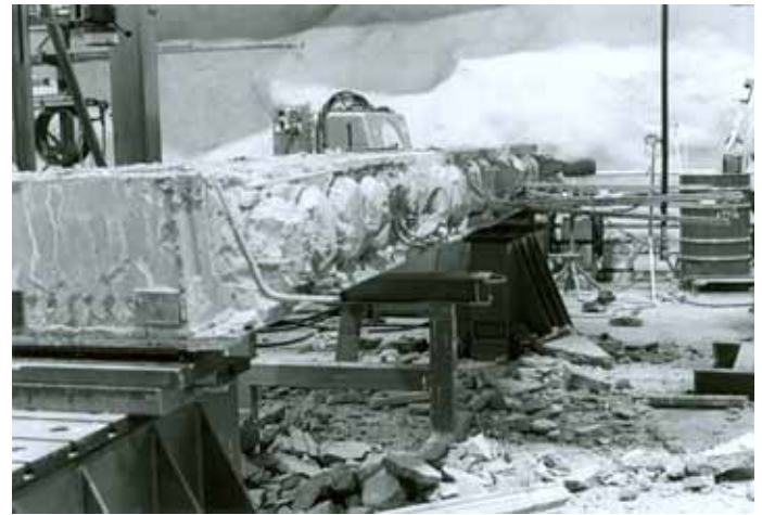
Fig. 16. Edge of middle beam after removing slab units 5–8.
