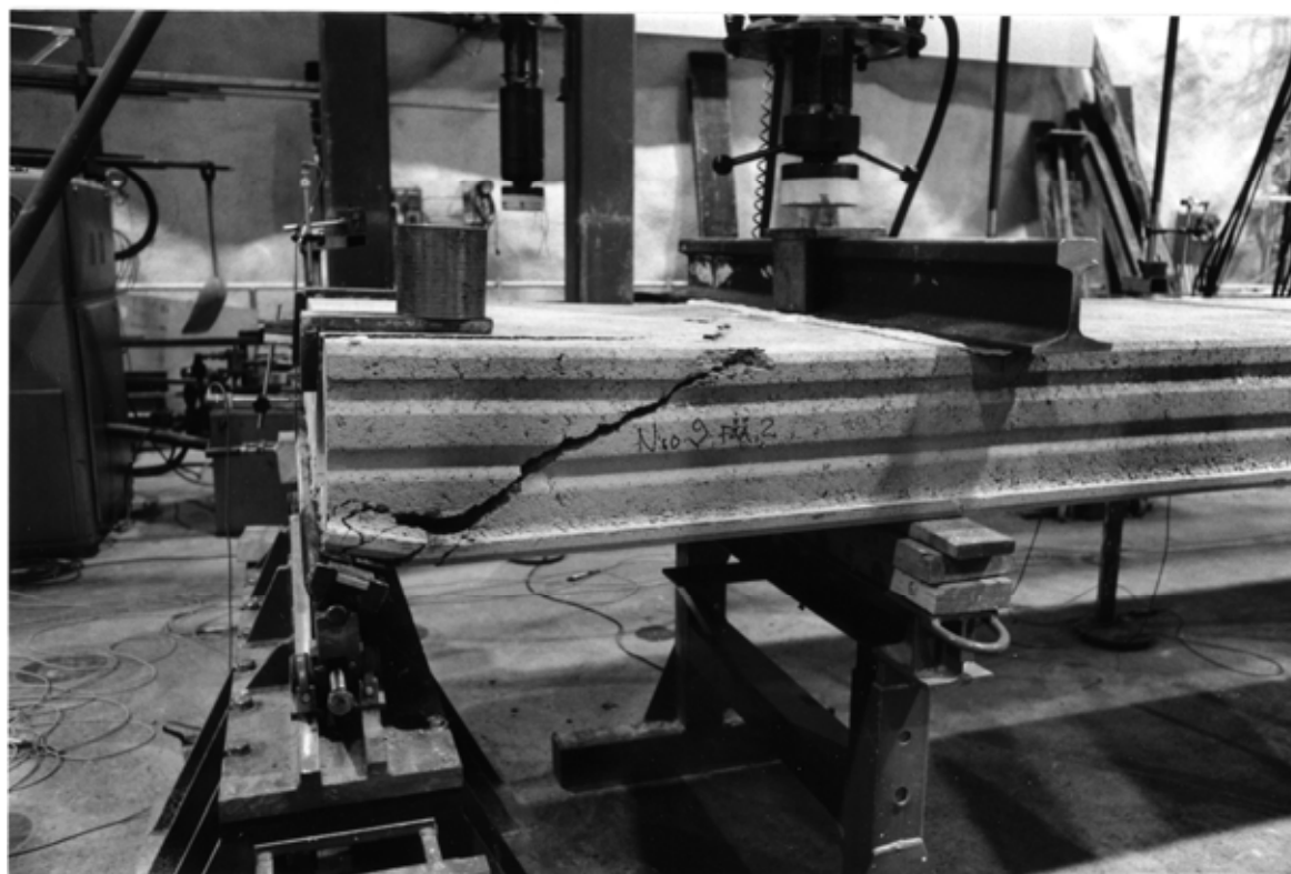
Fig. 20. The failure of the end 2 of the slab unit no 9 in the reference loading test.
