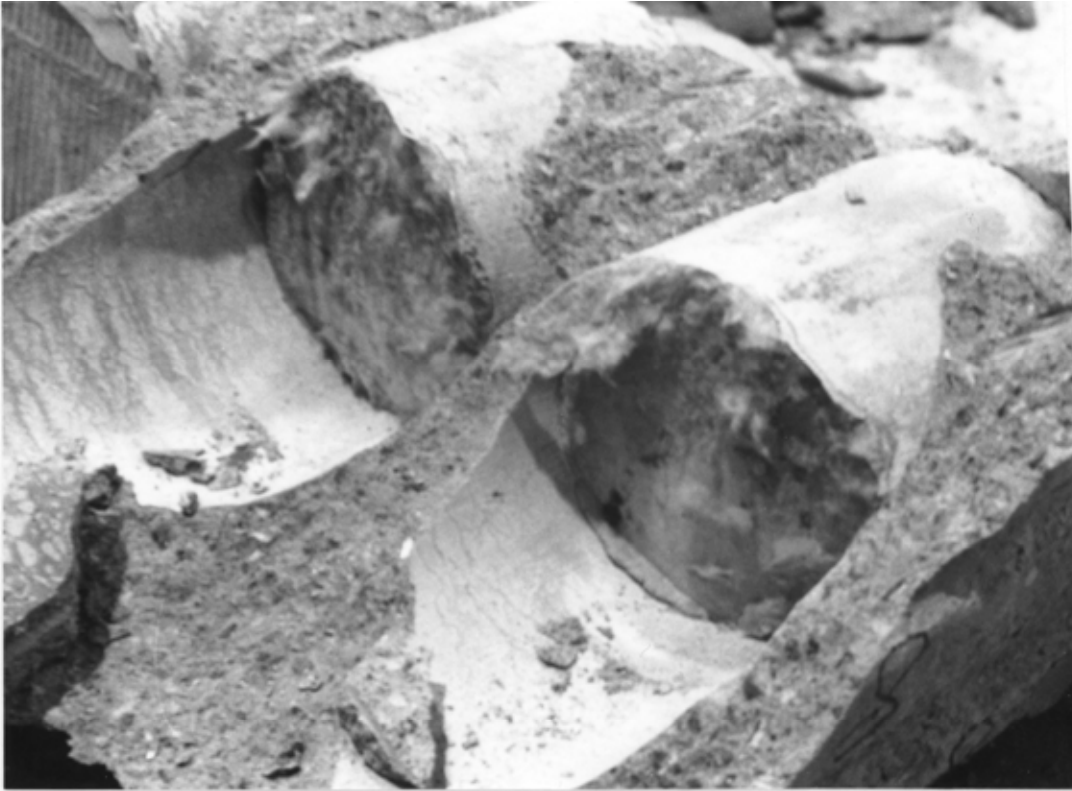
Fig. 20. Void filling at end of slab unit no 8 (upside down). Note that the concrete has filled the void completely.
