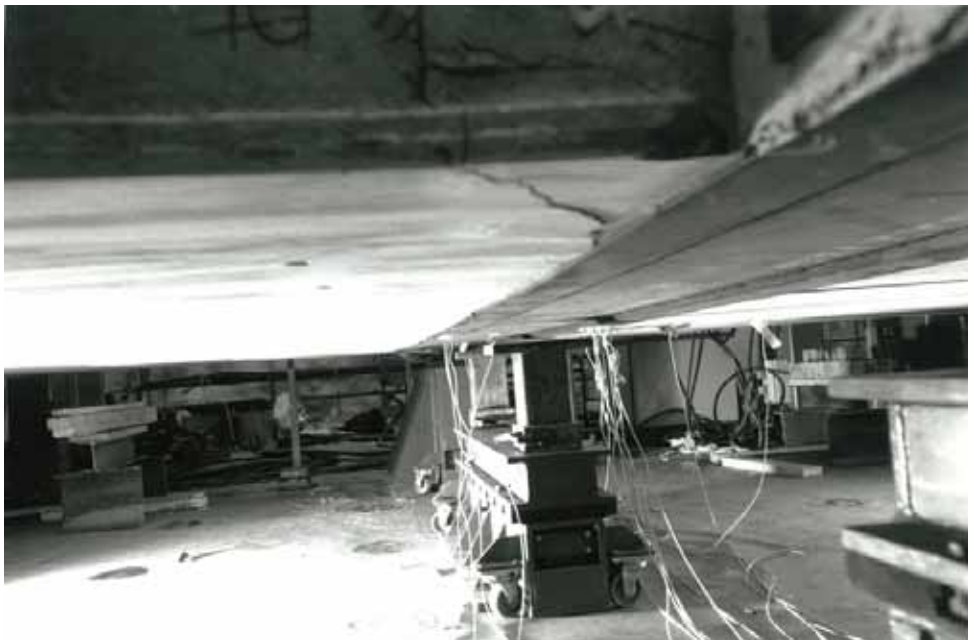
Fig. 22. Soffit of slabs 1–4 after failure.
