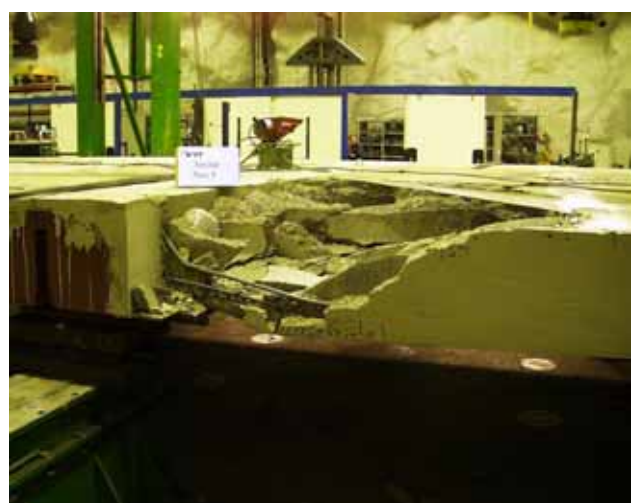
Fig. 42. End of slab 8 after removal of the top flange.
