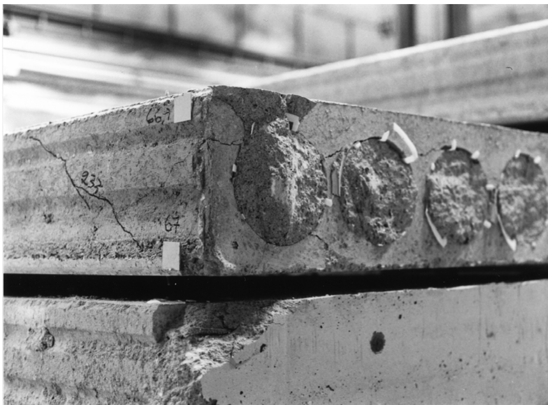
Fig. 17. Cracking of slab unit No. 6.
