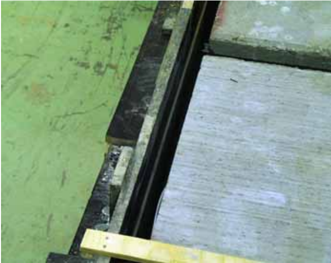
Fig. 7. End of floor before grouting.
