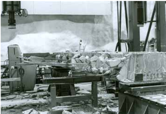
Fig. 15. Edge of middle beam after removing slab units 1–4.
