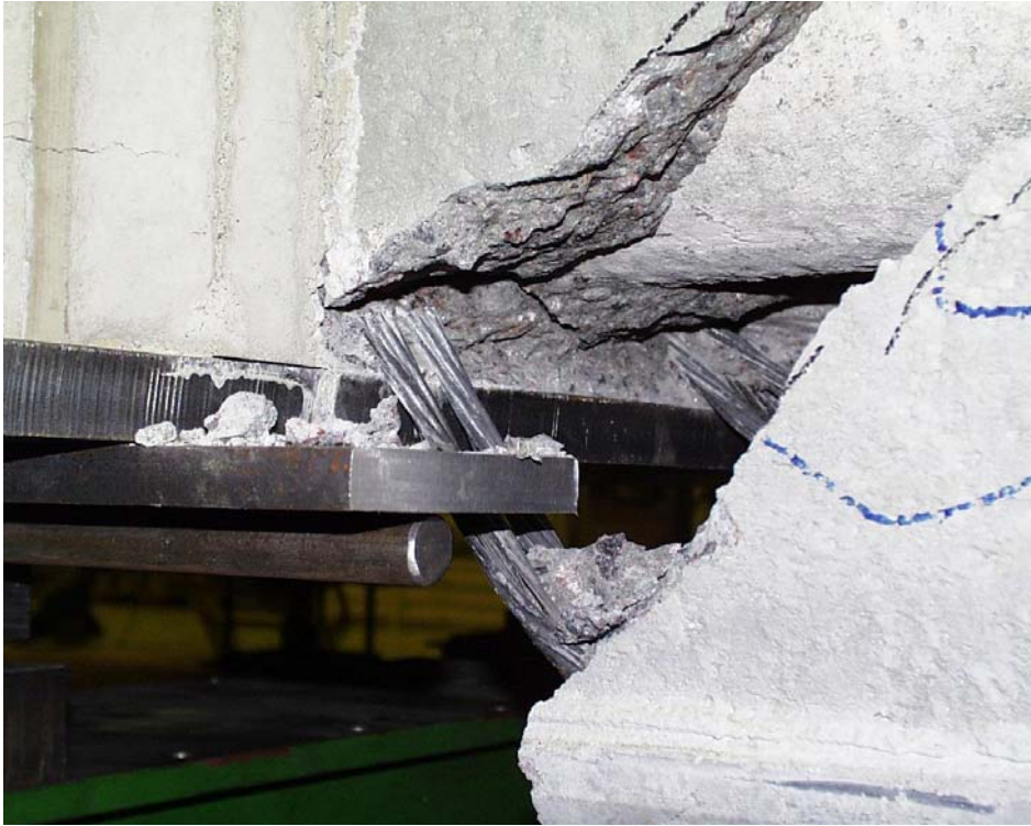
Fig. 43. Slab 12 after test.
