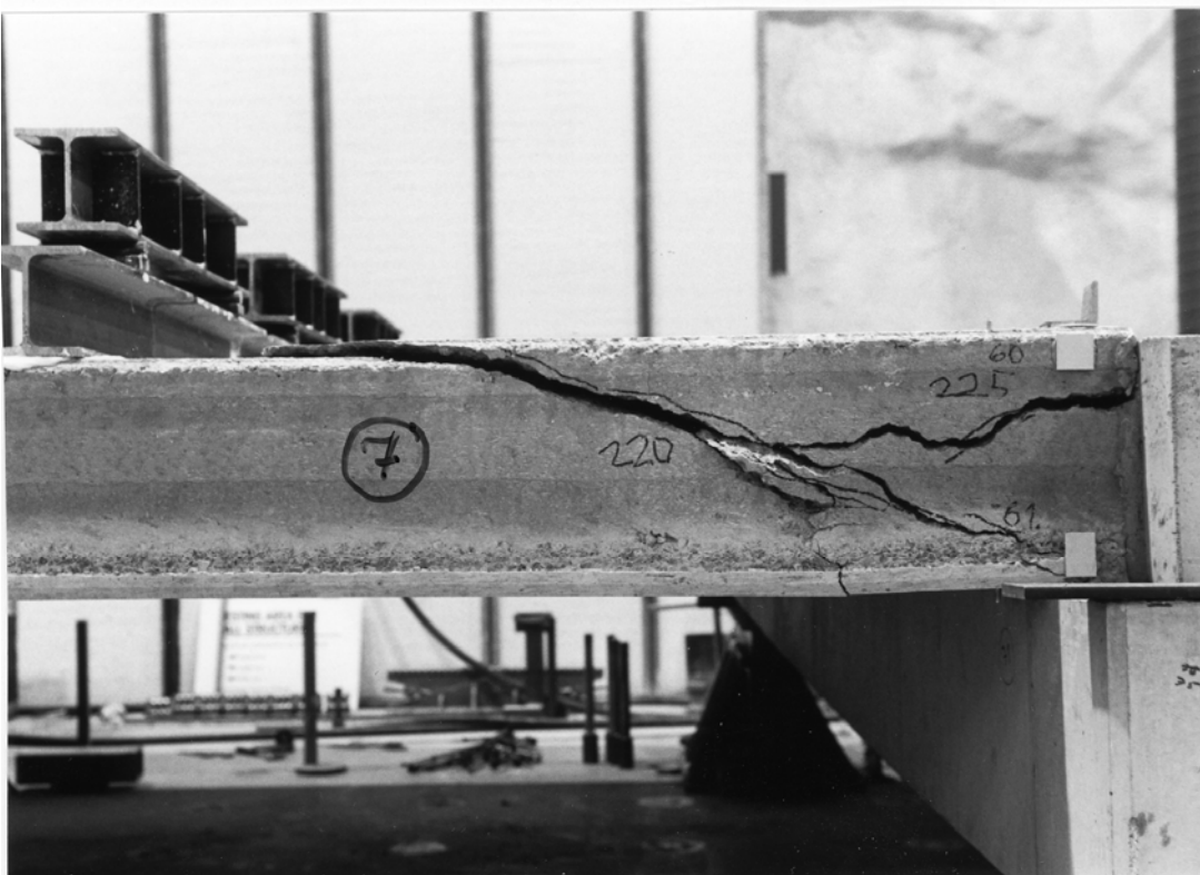
Fig. 8. Failure pattern of slab unit No. 7.
