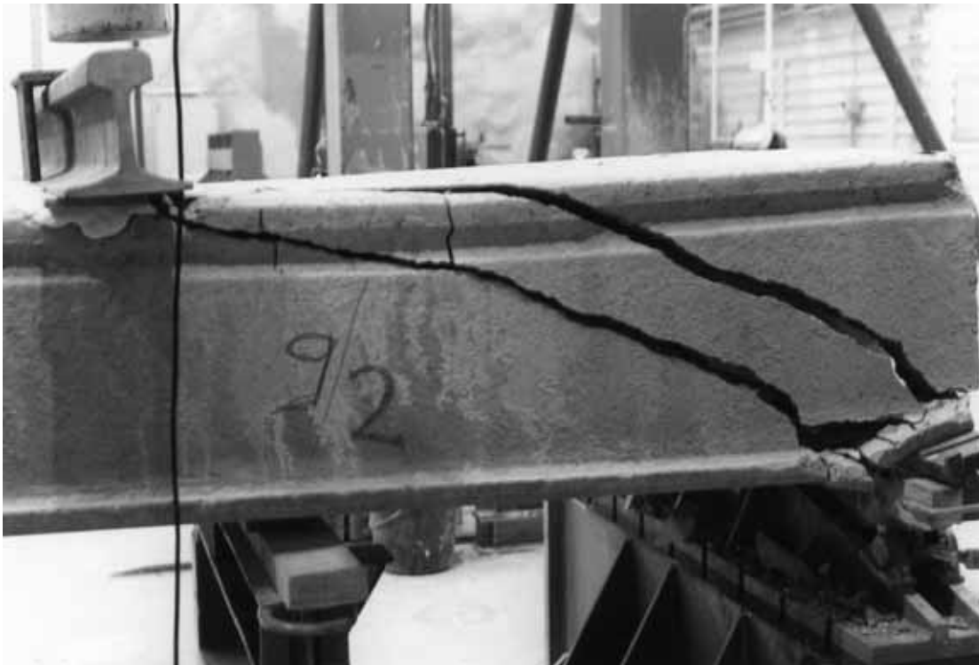
Fig. 31. Reference test R9/2. Failure pattern.
