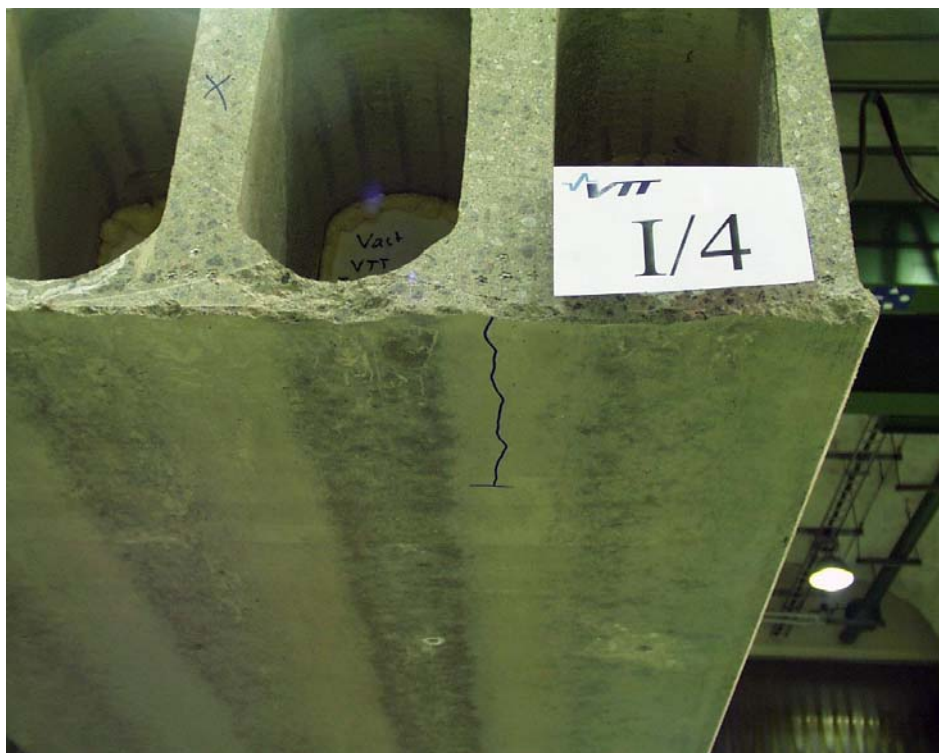
Fig. 5. Initial crack in slab 4.
