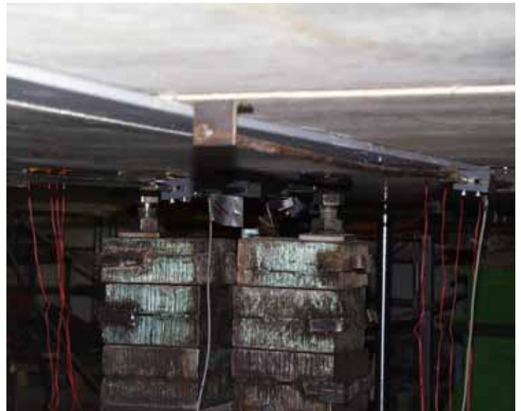
Fig. 13. Temporary support below mid-point of middle beam.
