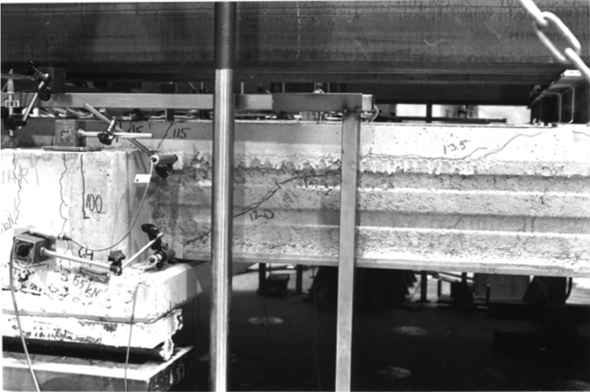
Fig. 10. The cracks in the longitudinal edge of the slab unit no 1, near the middle beam, at failure.
