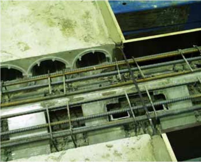
Fig. 1. Tie reinforcement at the edge of the floor.
