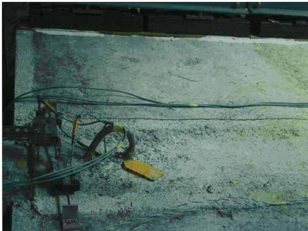
Fig. 3. A step between LB beam and slab 4.
