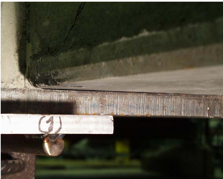
Fig. 44. Slab 1 after test.
