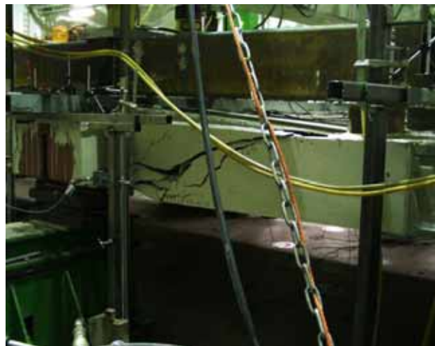
Fig. 26. Cracks in slab 8 after failure.
