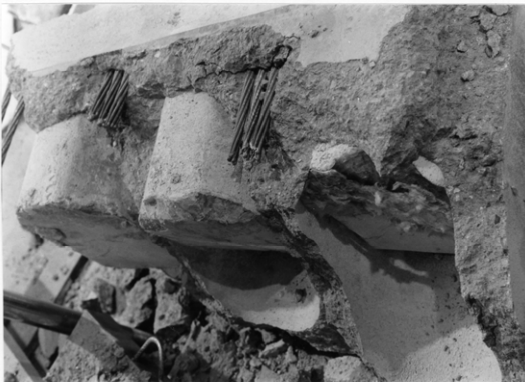
Fig. 8. Concrete in hollow cores. Note the proper filling.
