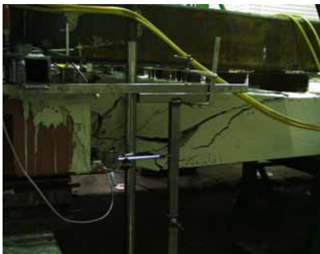
Fig. 27. Cracks in slab 8 after failure.
