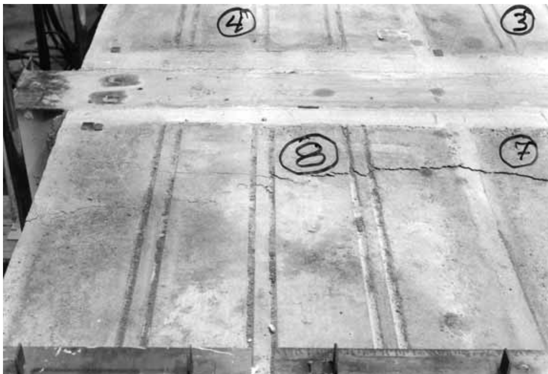
Fig. 21. Top surface of slab unit 8 after failure.
