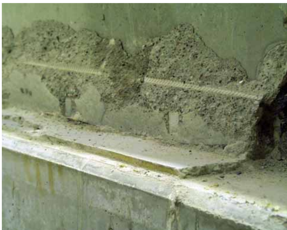
Fig. 28. Cast-in-situ concrete below slab end. Good bond with beam, weaker bond with slab.
