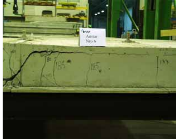
Fig. 32. Cracks in eastern tie beam after failure. Slabs 5, 6 and 7. The red colour and letter A refer to an initial crack.
