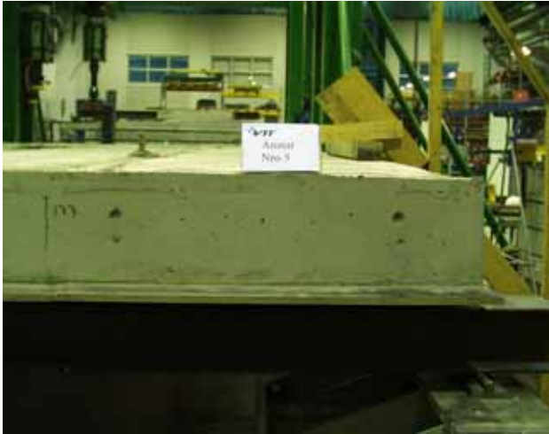
Fig. 31. Cracks in Eastern tie beam after failure. Slabs 5 and 6. The red colour and letter A refer to an initial crack.
