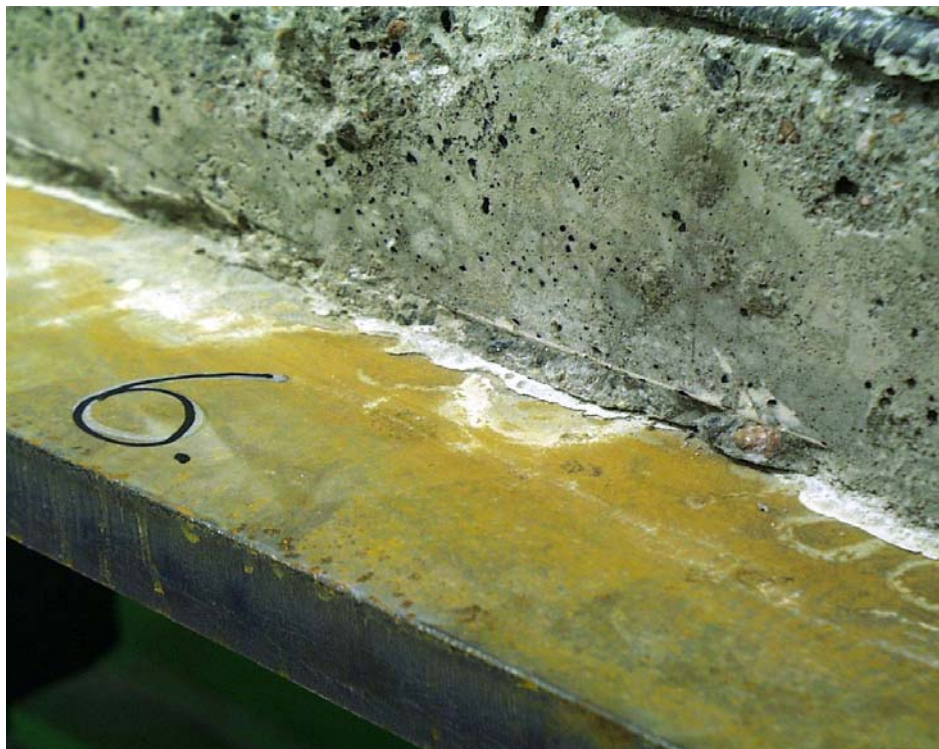
Fig. 57. A detail of grout below slab 6.
