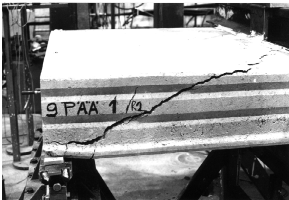
Fig. 14. The failure of the end 1 of the slab unit no 9 in the reference loading test.
