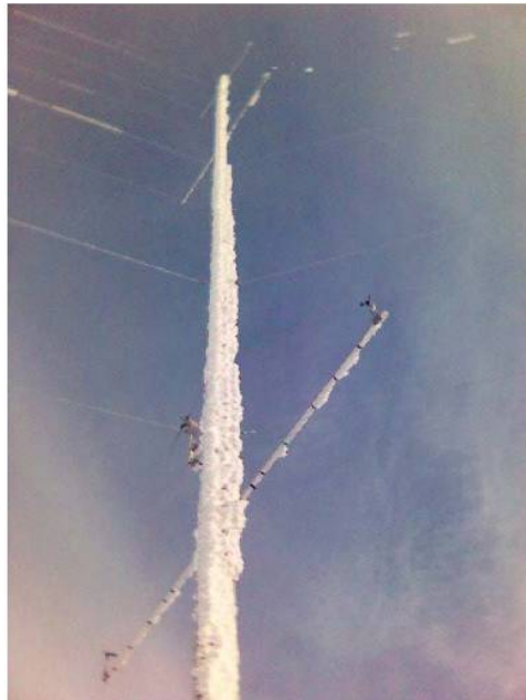
Figure 3. Meteorological tower with heavy icing.
