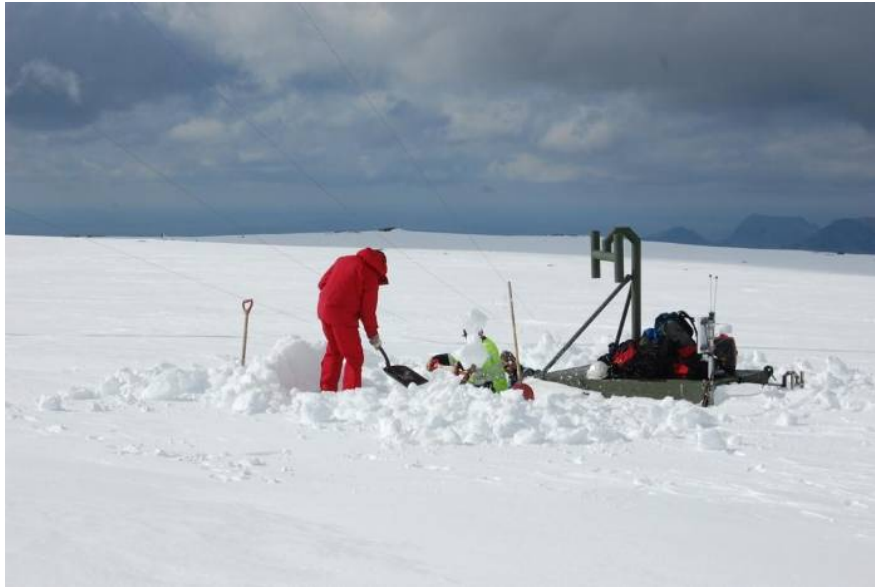
Figure 6. Accessing power system in a remote location. The whole structure apart from the air inlet to the engine has been buried. Photo credit: Lars Tallhaug, Norway.
