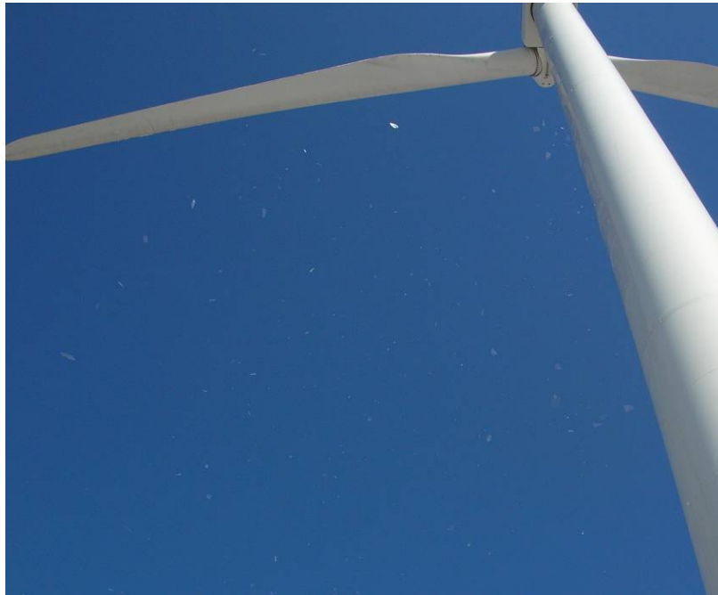
Figure 2. Ice falling or being thrown off a wind turbine poses a safety threat to turbine maintenance staff and depending on turbine siting, the general public. Photo credit: Jeroen Van Dam, USA.
