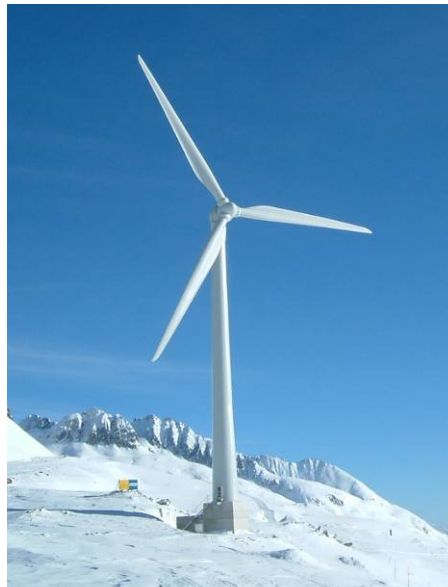
Figure 9. Turbine in Gütsch Switzerland is built on a ~10 meter concrete foundation with two levels of access to the turbine base and storage for extra turbine equipment. Photo credit: Markus Russi, Switzerland.
