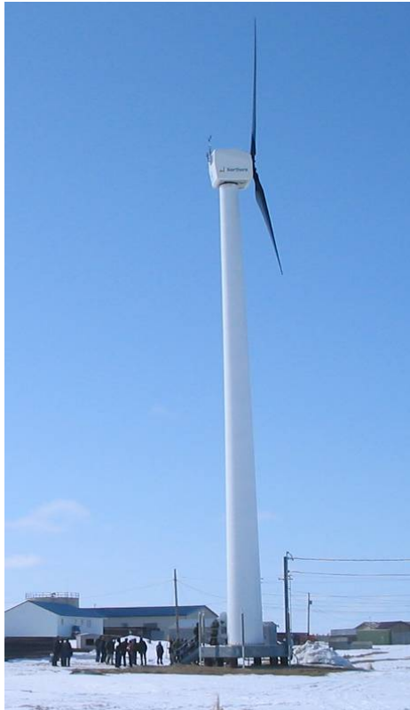
Figure 8. The Northern Power Northwind 100 allows service personnel to climb inside the tower and perform all general turbine maintenance from inside the nacelle. Photo credit: Ian Baring-Gould, USA.
