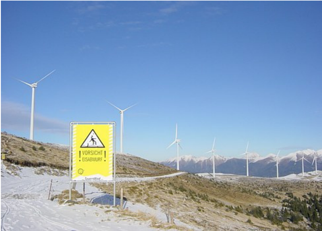
Figure 28. Warning against shedding ice fragments at Tauernwindpark in Austria. Photo from http://www.tauernwind.com .
